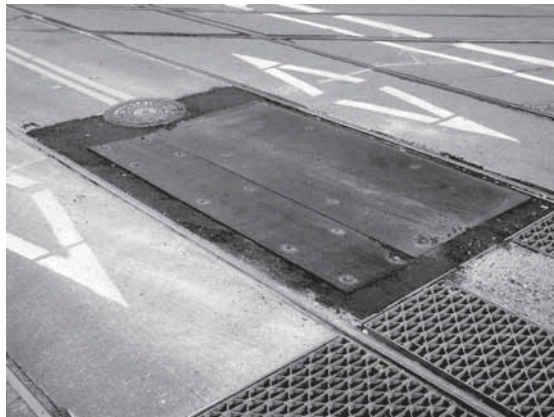
This construction plate lacks required non-skid coating.
