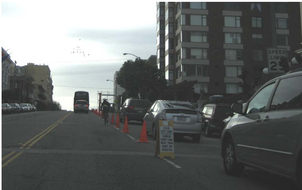
Figure 1: Lane Assignment Sign on westbound Broadway between Buchanan and Webster Streets. Sign reads “SSH Left Lane / Hamlin Right Lane Must turn right on Webster”
