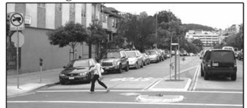
▼ A pedestrian refuge island shortens the crossing distance
