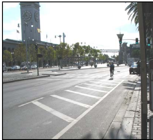
Figure 3. Cross-hatching at Beginning of "Floating Bike Lane" Treatment
