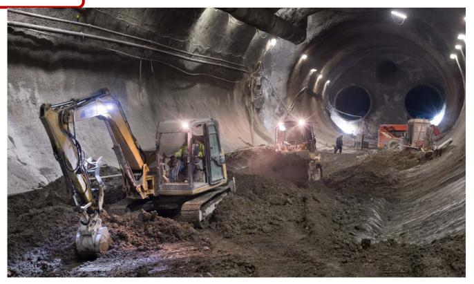
Work to complete excavation of the Chinatown station cavern is in its final stretch, with workers now removing all material from the invert prior to installing a waterproofing membrane.
