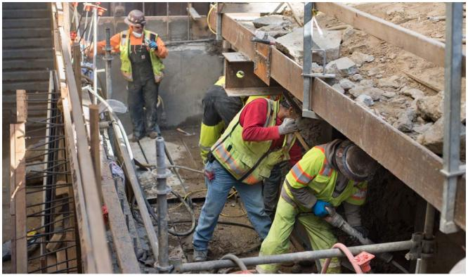
Workers chip away at concrete surrounding the tops of reinforced piles adjacent to the emergency egress staircase east of Stockton at O'Farrell.
