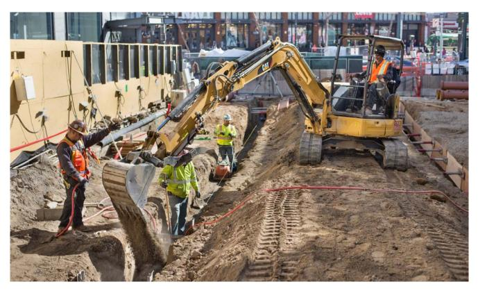
Sewer pipes and other utilities are being installed just above the buried roof deck of the Union Square/Market Street Station's south concourse, between Ellis and O'Farrell.
