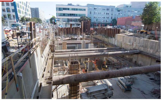
Looking south from Clementina, the temporary roof deck of the Yerba Buena/Moscone Station headhouse has been removed, allowing for construction of the final upper levels of that structure.
