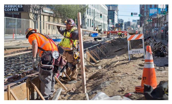
Two carpenters work on concrete form reinforcing for the base slab of the 4th and Brannan surface station.
