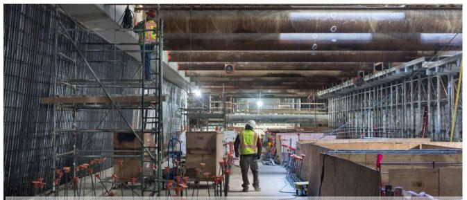
Looking south inside the Union Square/Market Street station box, crews have erected scaffolding and built concrete forms on the west side of the station's exterior walls, and are finishing rebar cage construction on the east. 8
