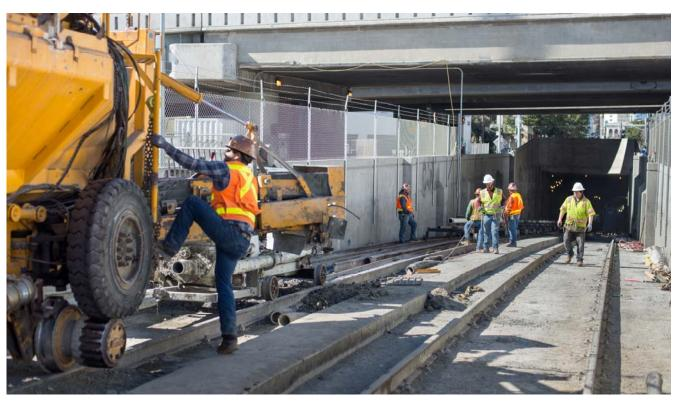
A crew emerges out of the tunnel portal following a concrete pour inside the southbound tunnel. Pipe sections mounted on carts used to pump concrete down the tunnel can be seen being cleaned out.
