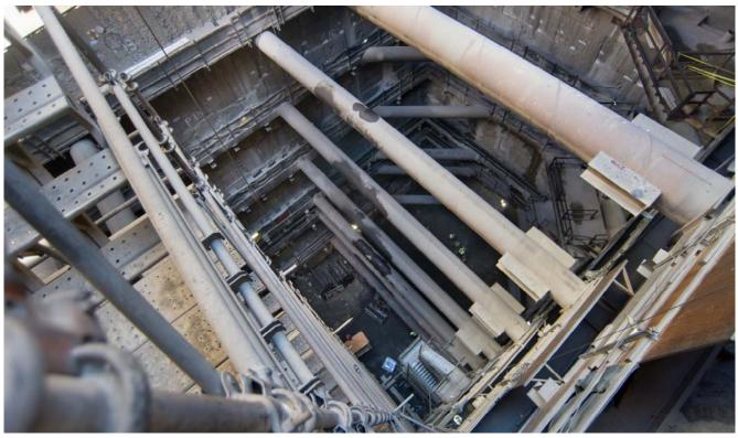
View looking 14 stories down into the Chinatown Station headhouse, with multiple rows and levels of steel struts reinforcing against soil pressure on the exterior slurry walls.
