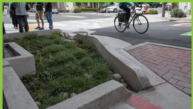
Example of a sidewalk 'raingarden' and permeable paving
