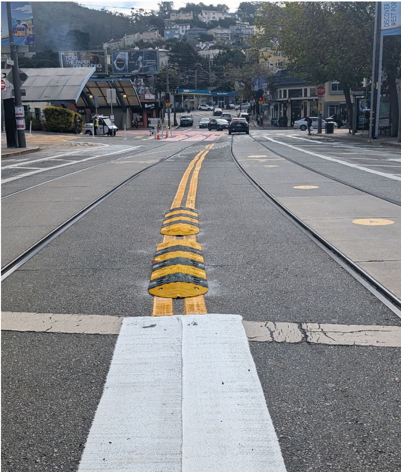
Centerline hardening on Ulloa Street
