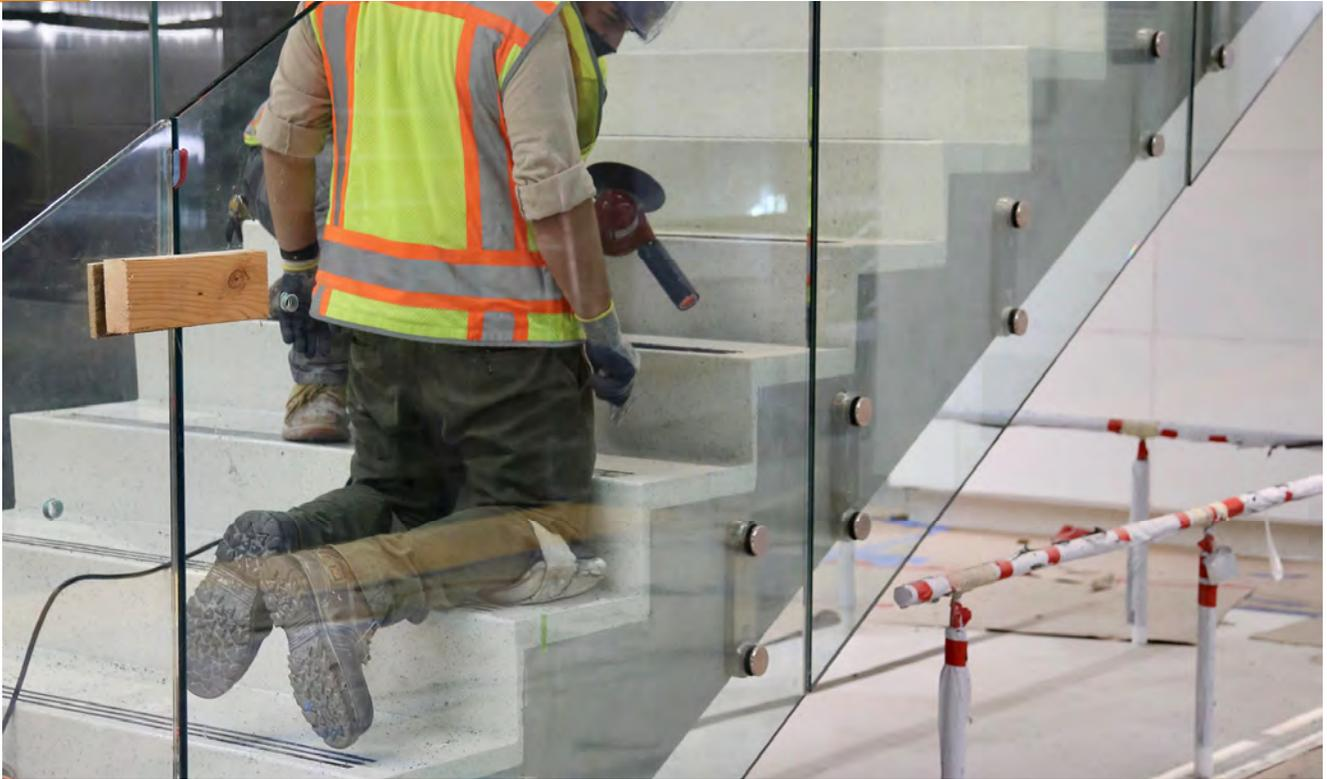
*Terrazzo staircase being finished and installed at Yerba Buena Station*
