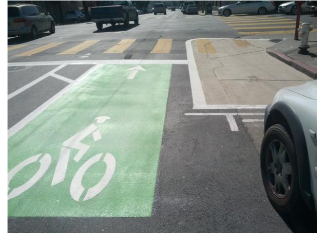
Painted Safety Zone and bicycle enhancement at Howard & 10 th (photo: Streetsblog)
