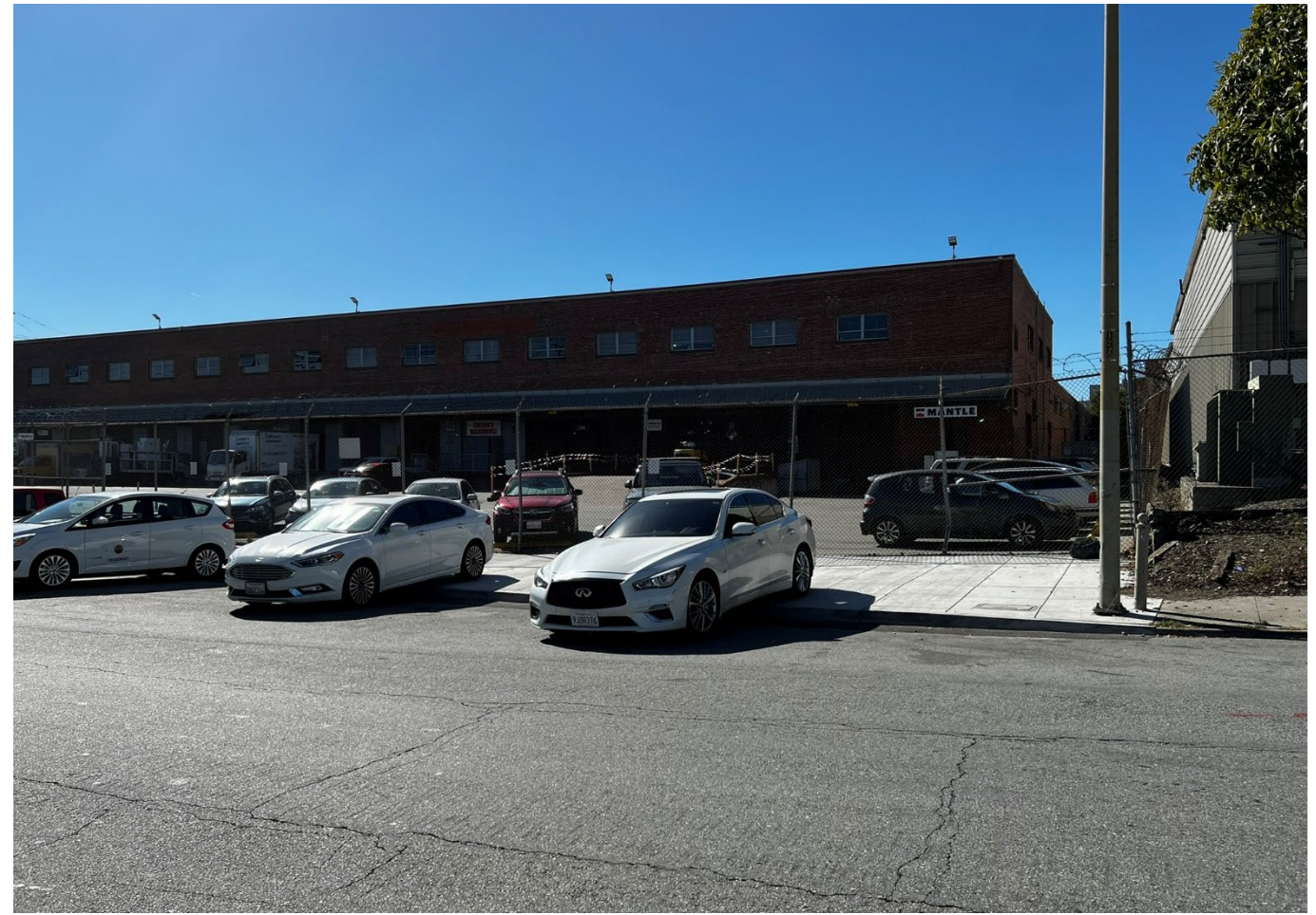
Connecticut Street post sidewalk construction
