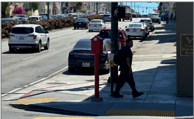
Pedestrian bulbs on 19th Avenue: Muni Forward installed 35 pedestrian bulbs along 19th Avenue, improving pedestrian safety on a state highway that functions as city street.
