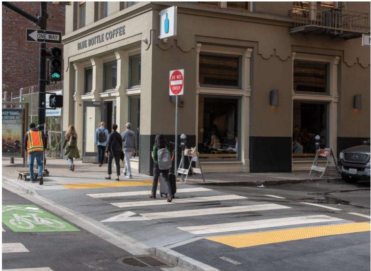
example of a raised crosswalk
