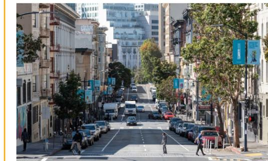
**Quick-Build Road Diets:** Quick-Build projects are reversible, adjustable traffic safety improvements that can be installed within months. Quick-Builds that remove a travel lane have been proven effective in slowing speeds in SF. For example, the 6th Street Pedestrian Safety Quick-Build resulted in a 21% decrease in 85th percentile speeds.
