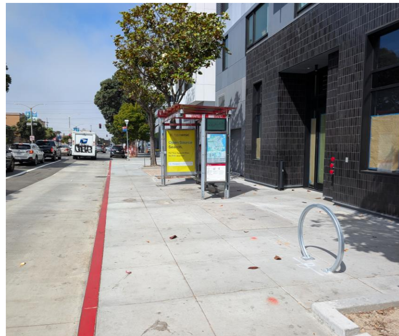
Recently completed Geary/6 th Avenue outbound bus bulb
