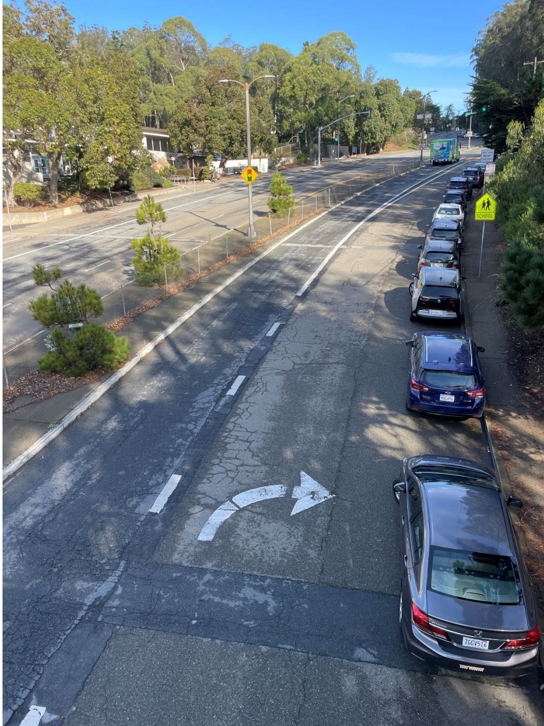
Clarendon Avenue at Ashwood Lane pedestrian bridge. Looking east uphill towards Panorama Drive
