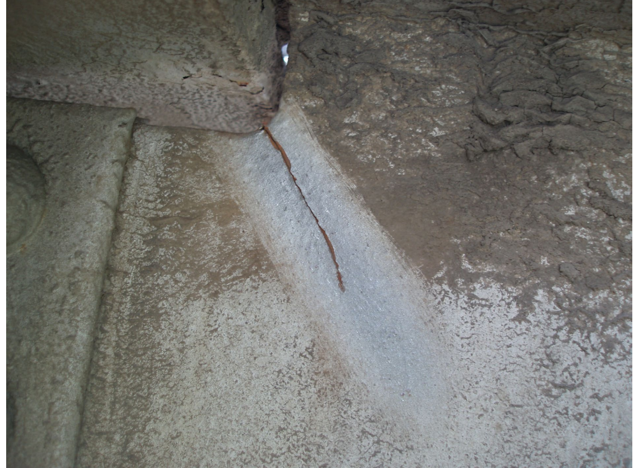
Deteriorated girders and fatigue cracks – Structural deficiencies noted in Caltrans Bridge Inspection – Impetus for rehabilitation in 2013
