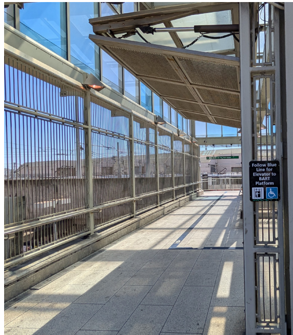
Elevated pedestrian walkway.
