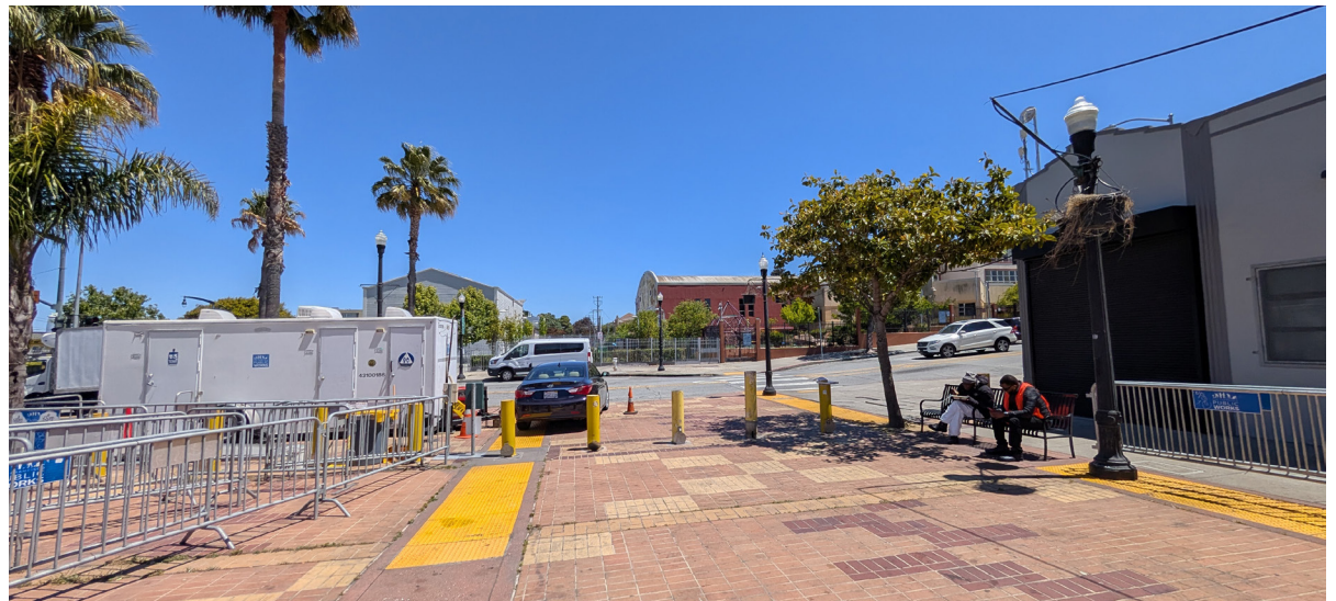
Bollards installed at Mendell Plaza to discourage vehicle access and portable restrooms.
