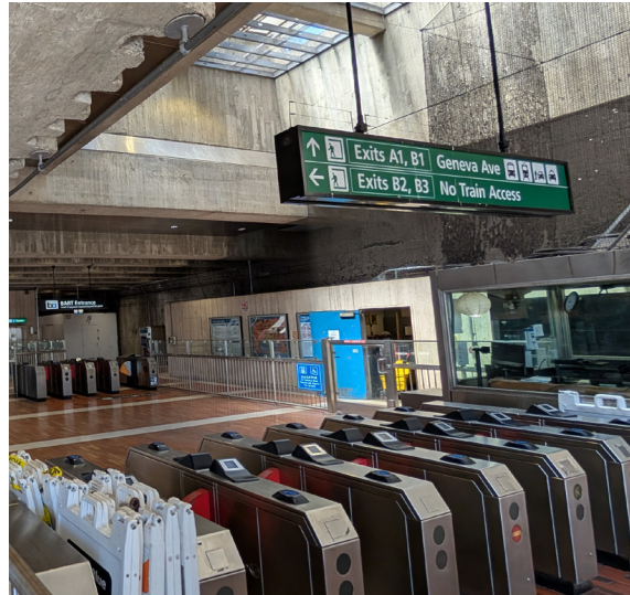
Wayfinding located at BART fare gates.
