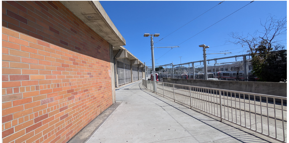
Pedestrian walkway along station edge.
