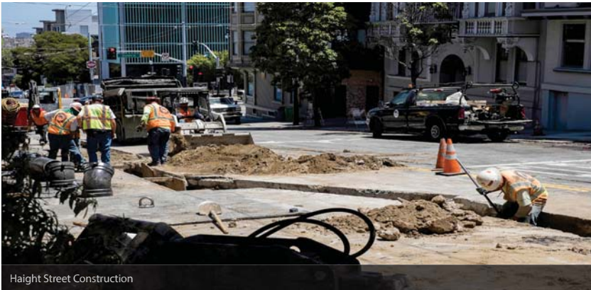
Haight Street Construction
