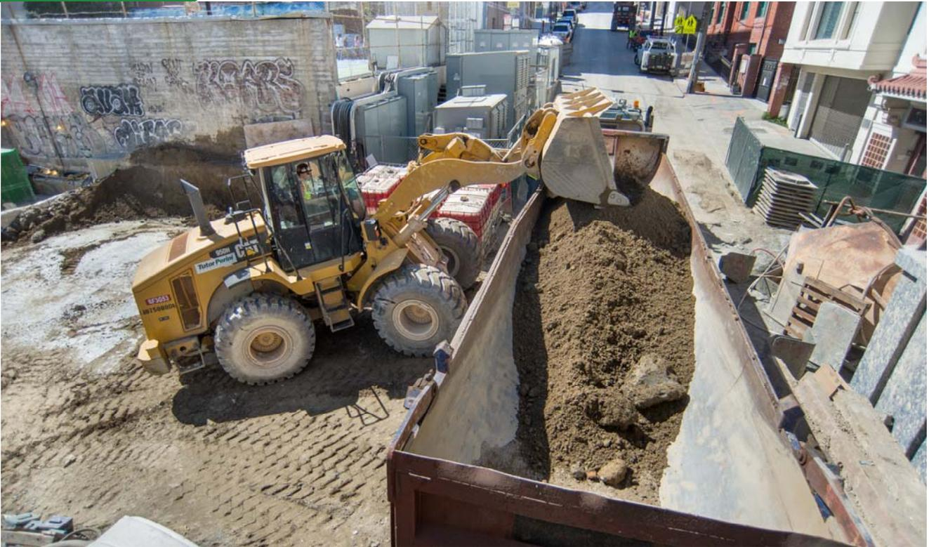
*As material excavated below is brought to the surface of the headhouse, a loader collects it and distributes the load evenly in trucks for transport offsite.*
