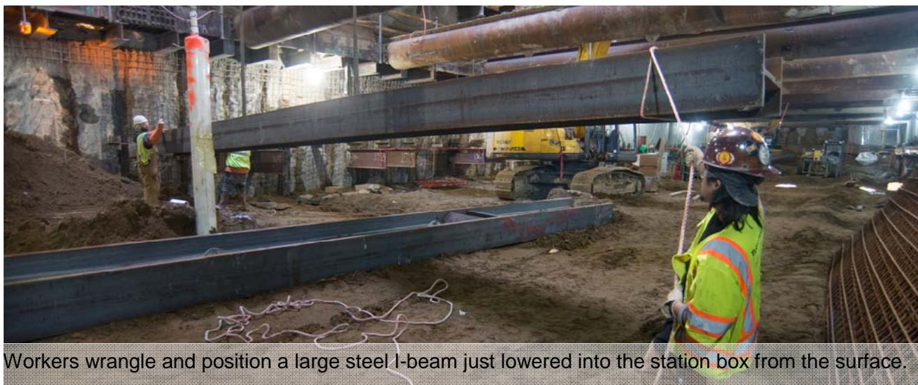
Workers wrangle and position a large steel I-beam just lowered into the station box from the surface.
