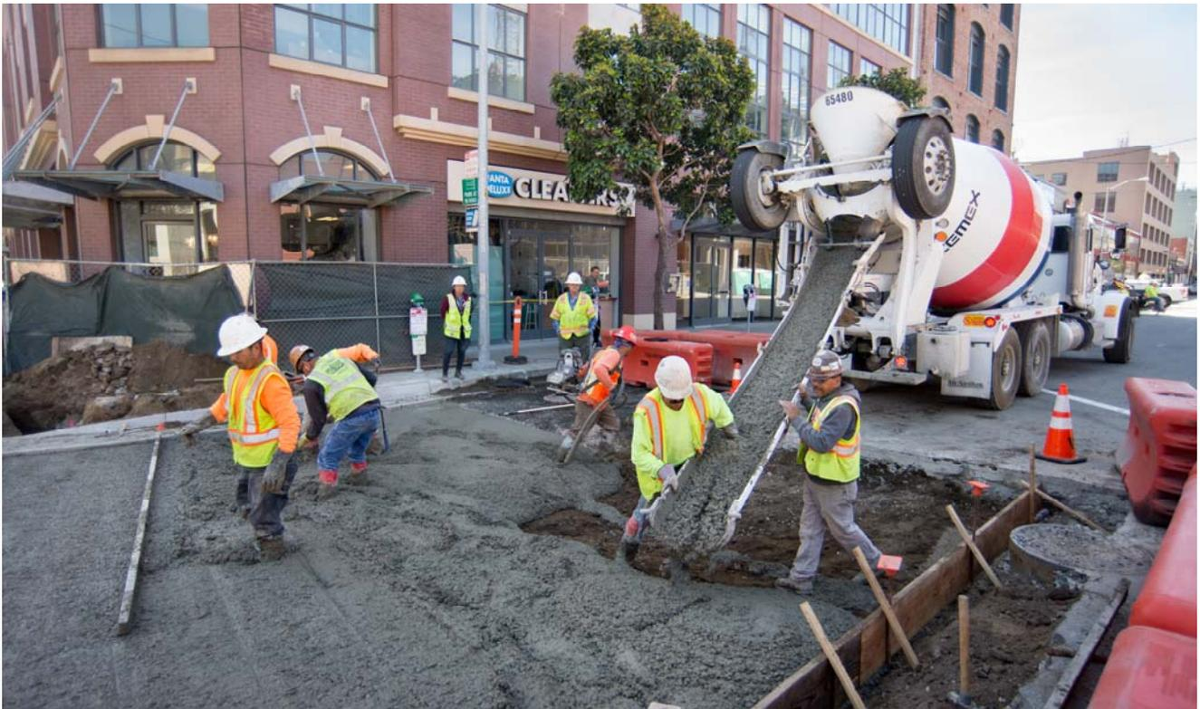
*A new concrete road foundation slab is being poured at the southwest corner of 4th and Bluxome.*
