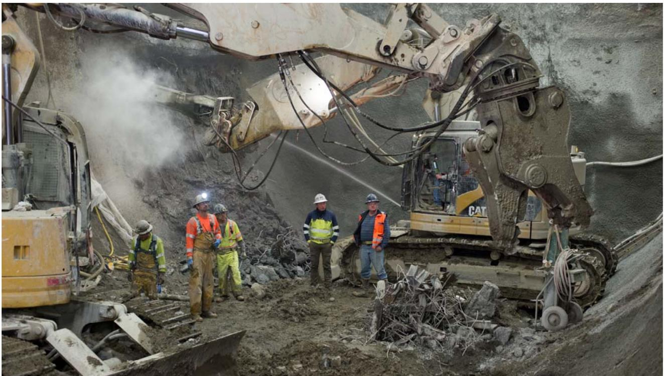
*Demolition jaws are moved into place to see how effective they are at removing reinforced shotcrete during excavation inside the cross-cut cavern area.*
