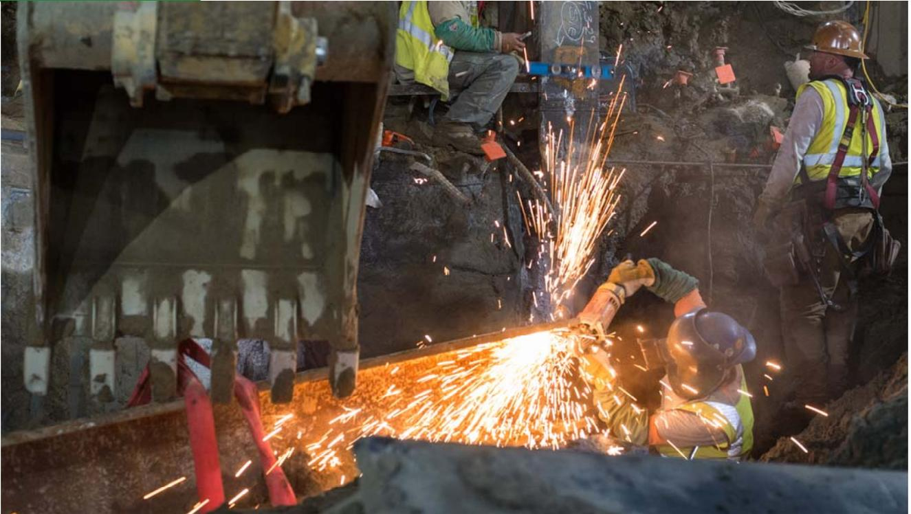
*A metalworker cleans up the ends of a large steel I-beam for welding, which will be used as a bracket at the south headwall, near O'Farrell.*
