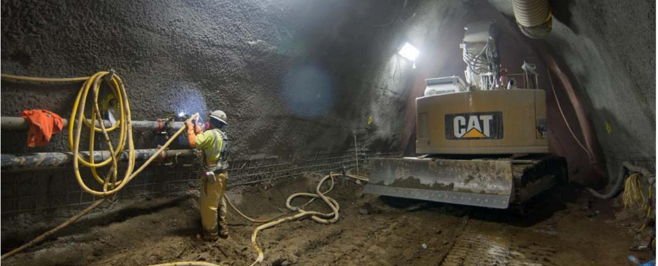
*A worker checks the air pressure on a hose inside the left side drift of the north platform cavern, while a large excavator fitted with a grinding wheel works away nearby.*
