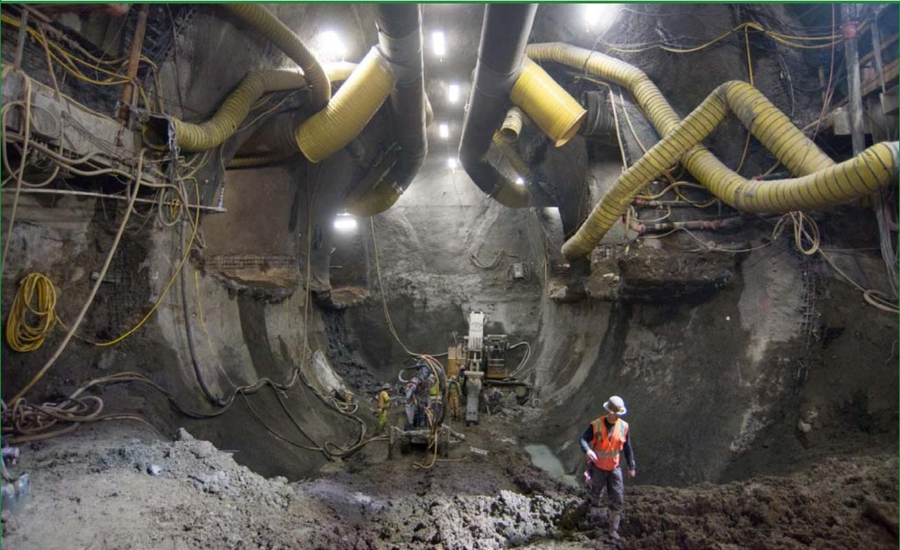
**Cover photo:** At the bottom of the tunnel portal ramp, the northbound and southbound tracks transition to the twin subway tunnels, curving outward slightly before running parallel to the Yerba Buena/Moscone Station just a block away. Workers have installed concrete forms to construct the remaining elements of the tunnel portal invert, and track foundations called plinths. **More photos can be found starting on page 36.**
