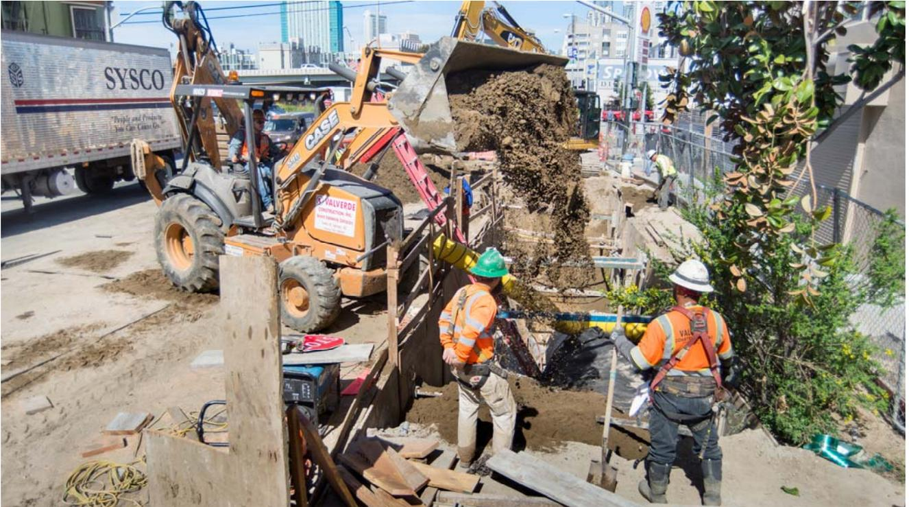
***A backhoe brings a bucket of soil to bury newly-installed sewer pipes between Welsh and Bryant, on the east side of 4th.***
