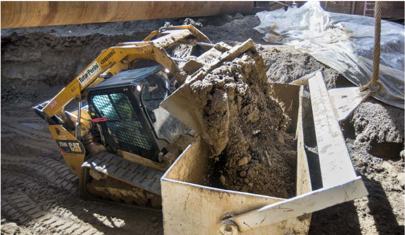
***A bobcat dumps soil excavated from inside the station headhouse into a large steel bucket used to lift material to the surface for transport offsite.***
