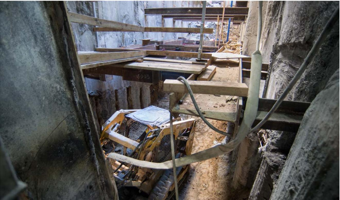
*A bobcat fitted with a jackhammer is used to remove excess concrete from exterior tangent piles, comprising the station's outer walls. In this area on the east side of the station box at O'Farrell, workers are excavating a future emergency egress stairwell.*
