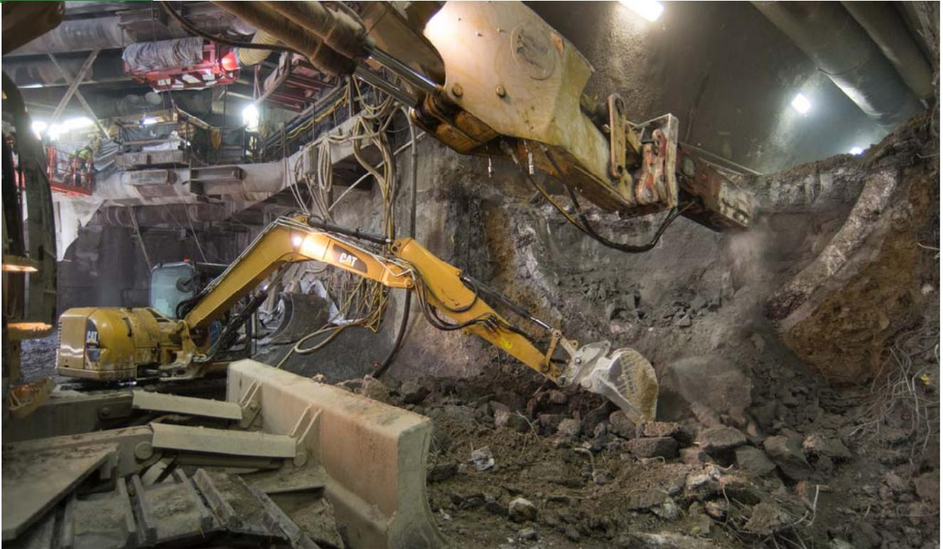
*The faint outline of remaining tunnel segment pieces can be seen as it is removed during excavation of the left side drift for the north platform cavern.*
