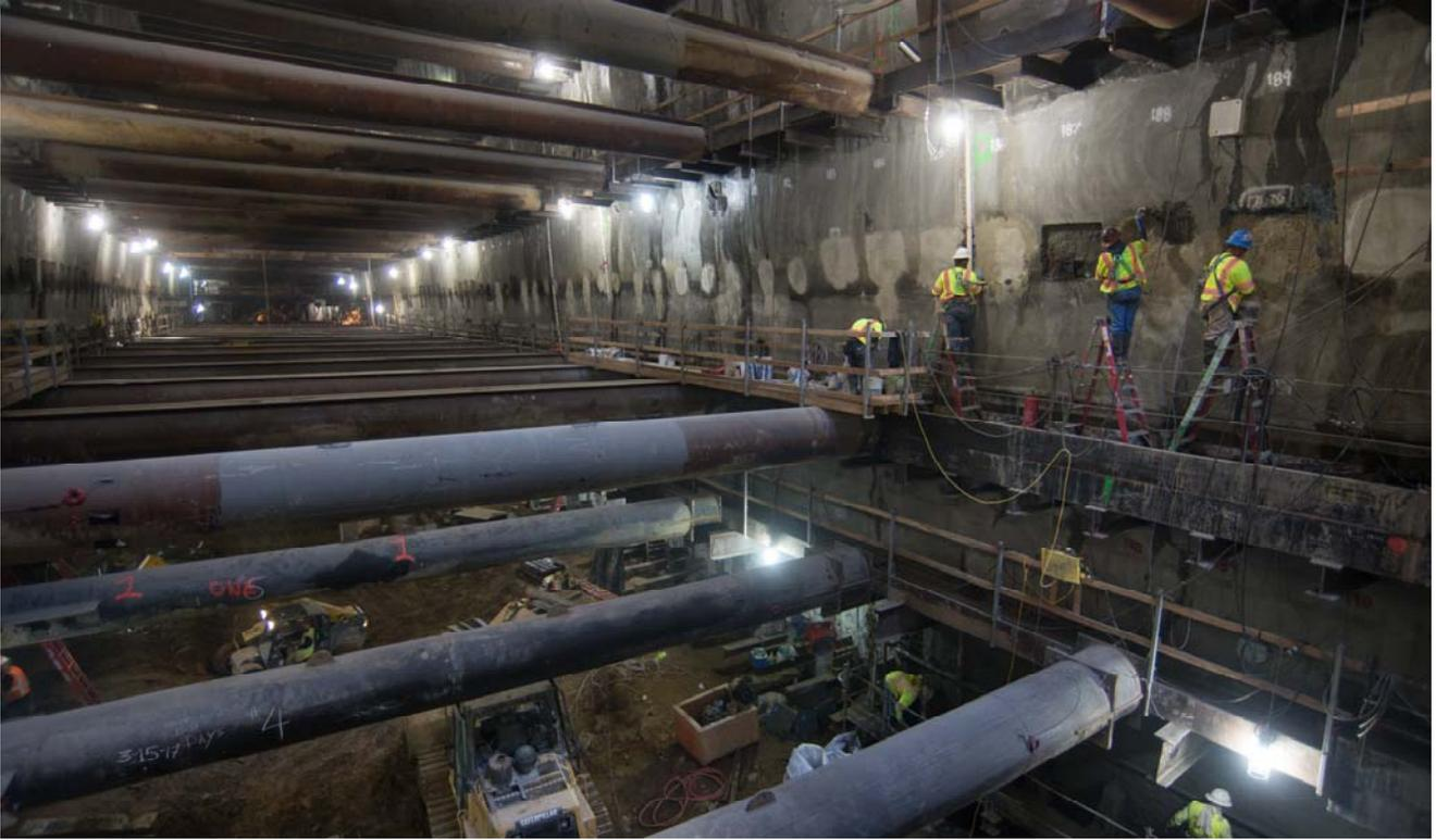
*A small crew applies patching to shotcrete on the west wall of the station box, while excavation and shotcrete installation work occur below.*
