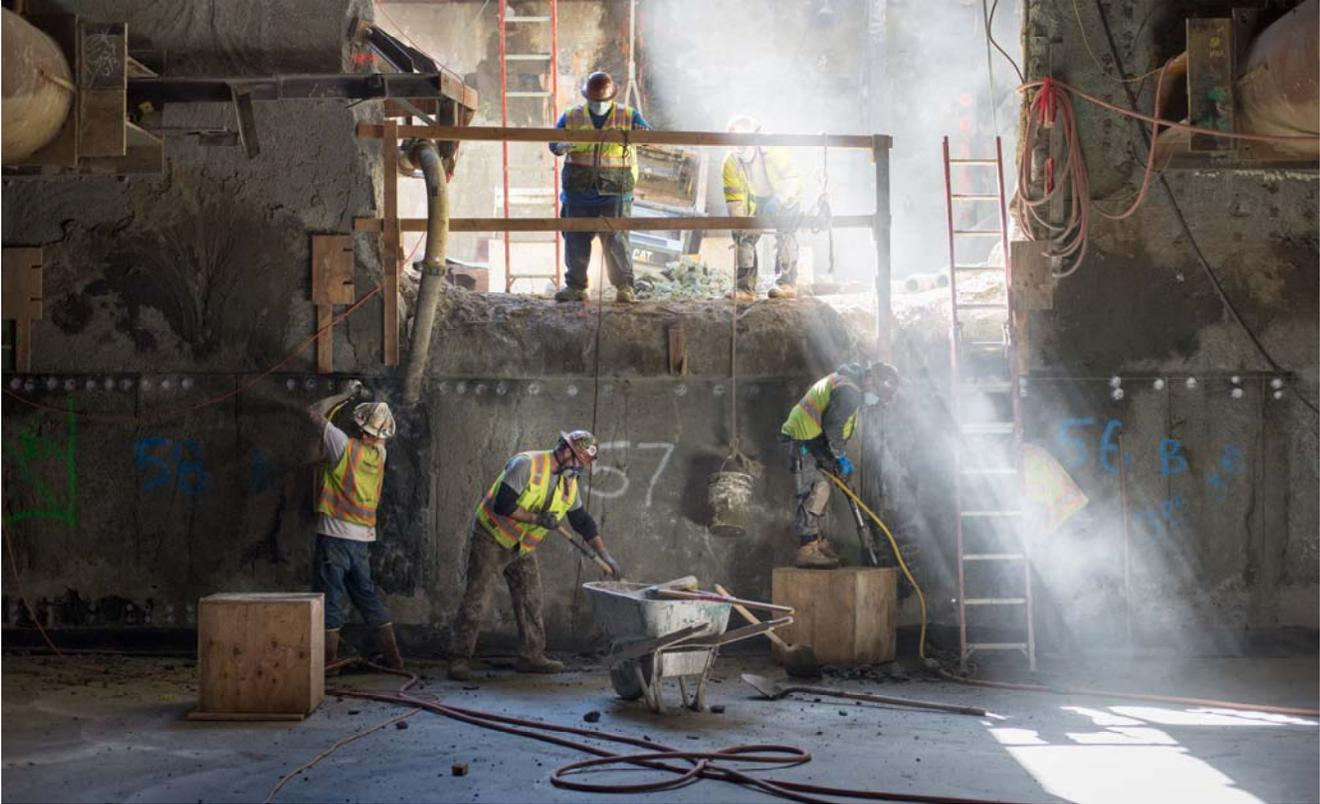
*Workers chip away at the bottom of the access portal to the station box from the head-house, prior to constructing the station box platform level invert in this section.*
