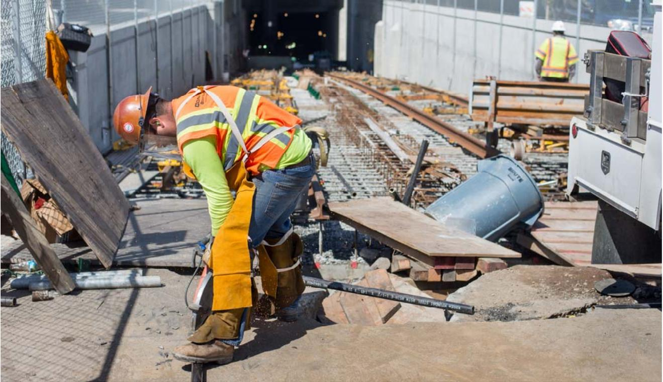
*Sections of small steel pipe are cut as part of the final push to construct the remaining elements of the invert slab for the tunnel portal.*
