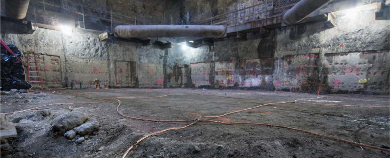
*Copper grounding wire has been placed at the south end of the Chinatown station headhouse following the completion of excavation and grading work, there.*
