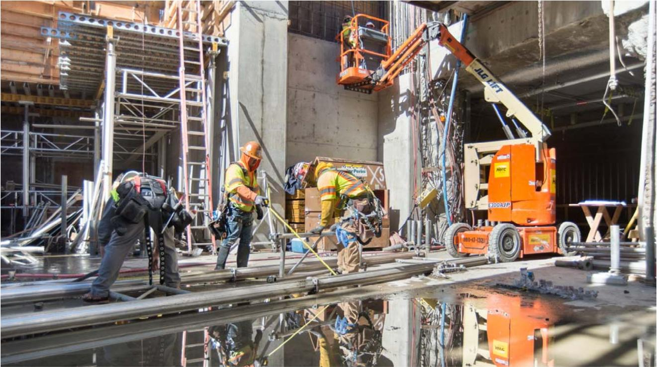
***Reinforced vertical scaffolding is assembled inside the headhouse, near the portal into the station box concourse. This scaffolding will eventually support roof deck formwork.***
