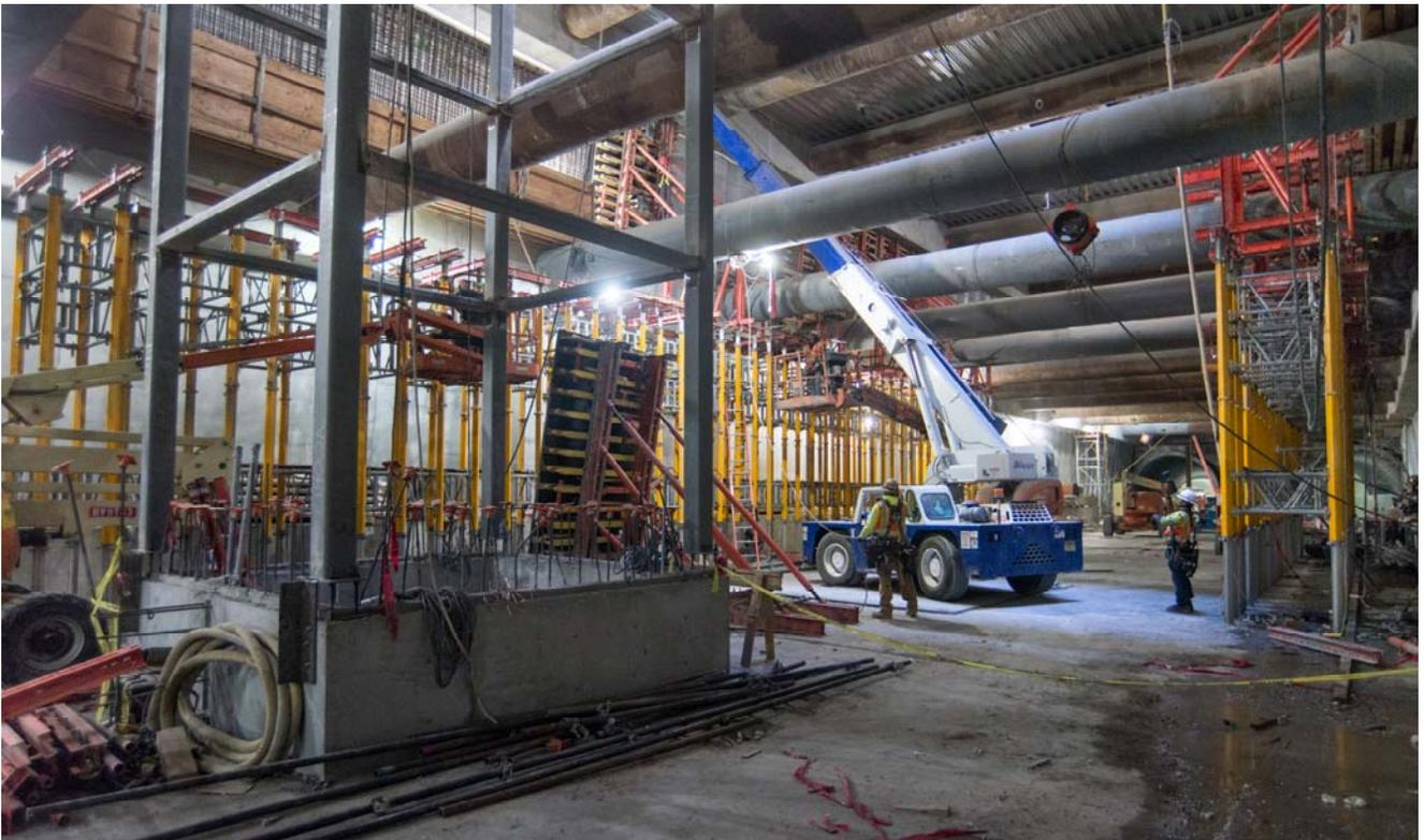
***Light beams in through a street-level access portal high above just north of O'Farrell as workers install sections of concrete forms just above the platform level inside the Union Square/Market Street station box.***
