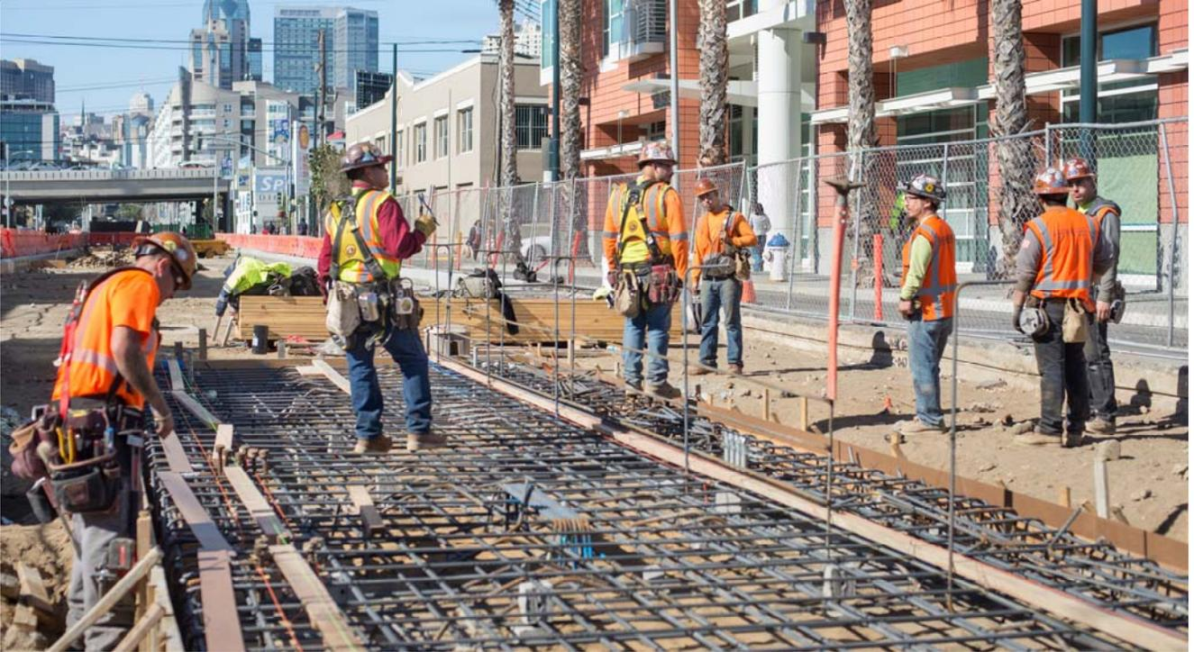
***Workers use steel wire to join long pieces of rebar at the 4th and Brannan station site, and wooden stakes with snap lines maintain level construction.***
