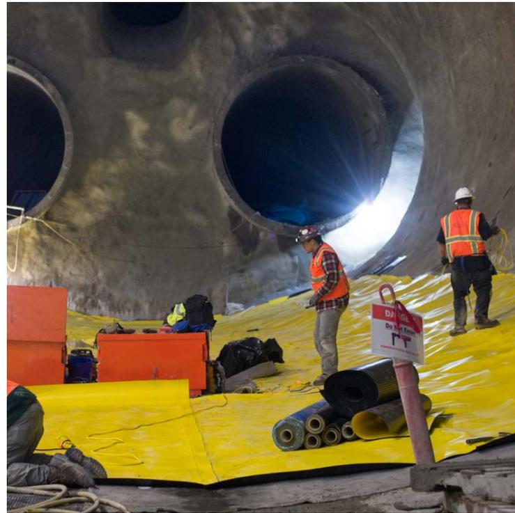
3 Sheets of waterproofing are installed and sealed into one huge sheet
