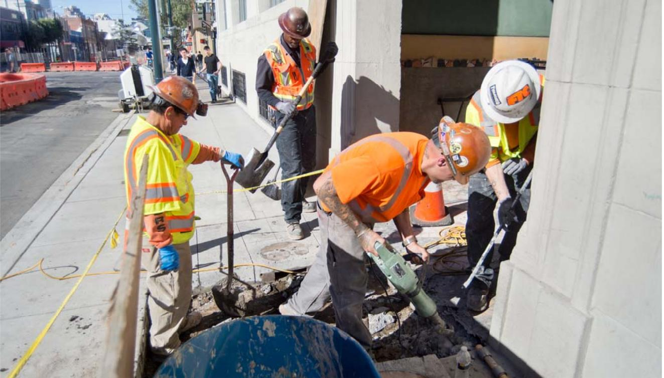
*A section of sidewalk is removed from the entry to 601 4th Street for replacement and as the contractor conducts sidewalk follow-up work on the east side of 4th Street.*
