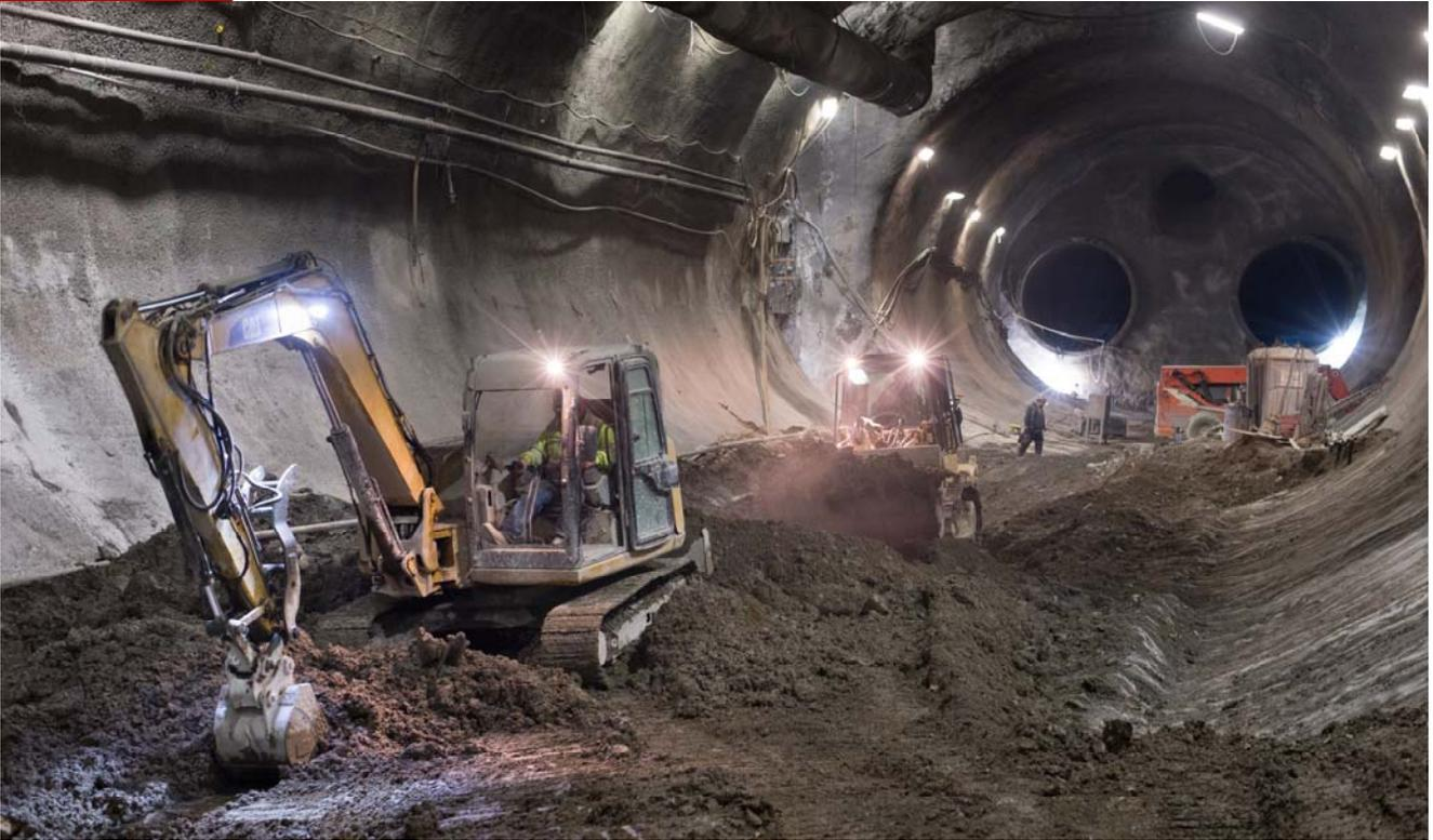
*Work to complete excavation of the Chinatown station cavern is in its final stretch, with workers now removing all material from the invert prior to installing a waterproofing membrane.*
