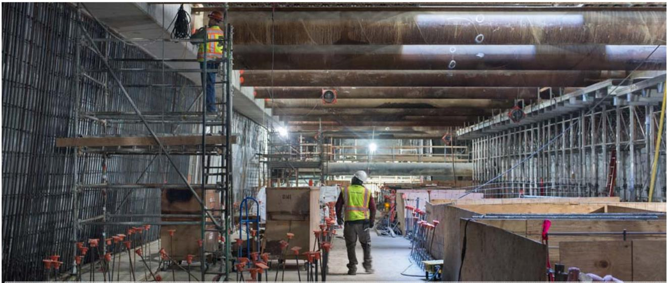
Looking south inside the Union Square/Market Street station box, crews have erected scaffolding and built concrete forms on the west side of the station's exterior walls, and are finishing rebar cage construction on the east.
