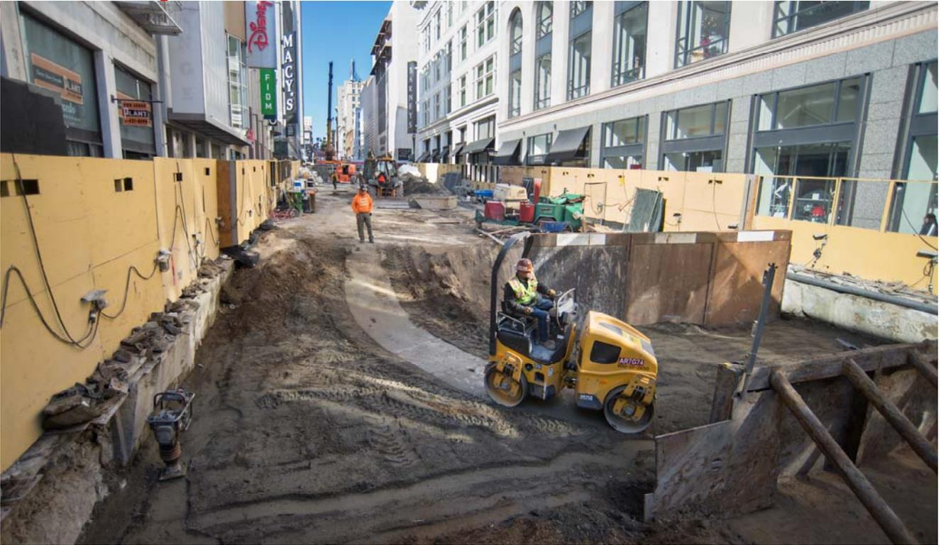
***Soil is compacted at the former access shaft just north of Ellis on Stockton over the south concourse, which has recently been permanently covered over with the completion of the last section of roof decking, there.***
