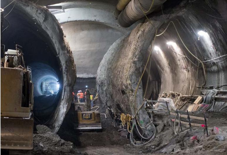
1 Excavation is completed and shotcrete separator walls are removed
