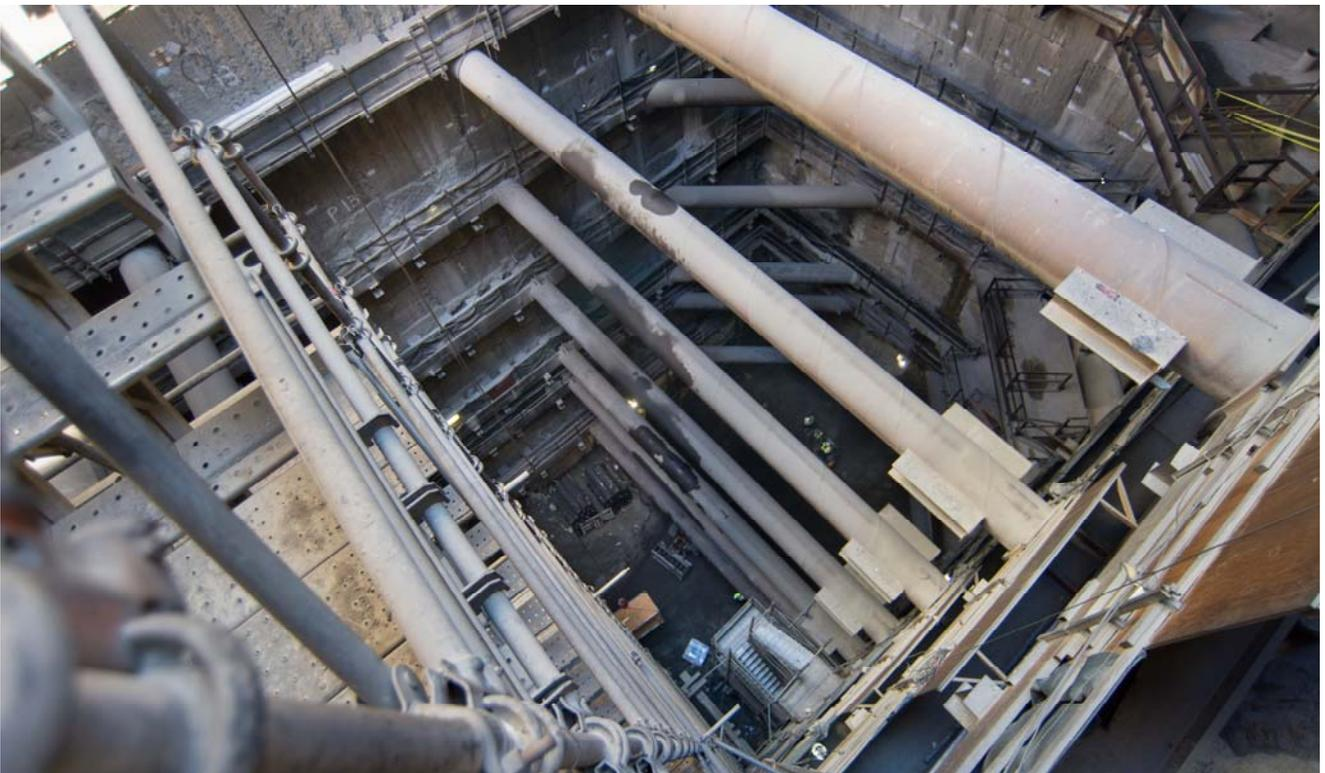
*View looking 14 stories down into the Chinatown Station headhouse, with multiple rows and levels of steel struts reinforcing against soil pressure on the exterior slurry walls.*
