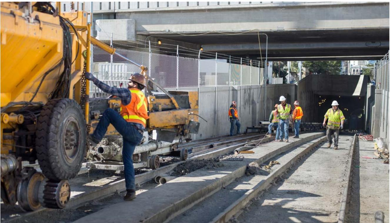
*A crew emerges out of the tunnel portal following a concrete pour inside the southbound tunnel. Pipe sections mounted on carts used to pump concrete down the tunnel can be seen being cleaned out.*
