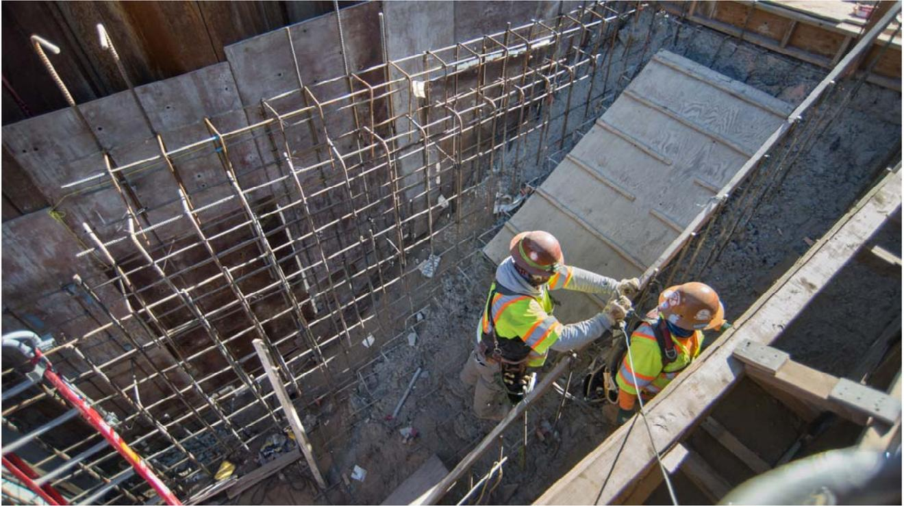
*Initial rebar cage assembly is under construction for the exterior walls of an emergency egress staircase at the southwest corner of the Yerba Buena/Moscone worksite.*
