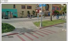
The SFMTA will test measures to slow bicycles as they approach pedestrian crossings. For instance, SPEED REDUCTION STRIPES use narrow strips of paint or textured pavement that can be both seen and felt. If effective, these could be rolled out throughout the project area.
