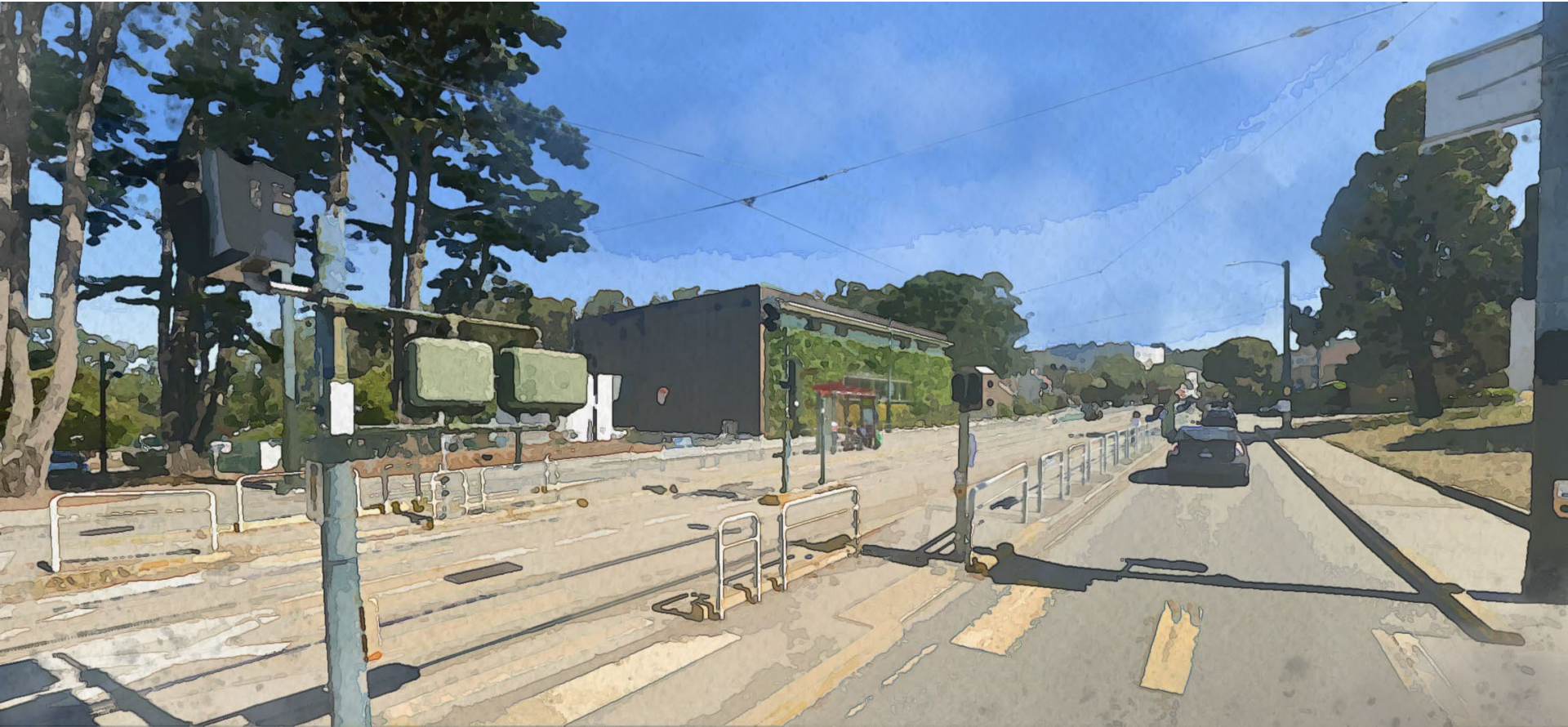
St. Francis Circle station– Existing Conditions
