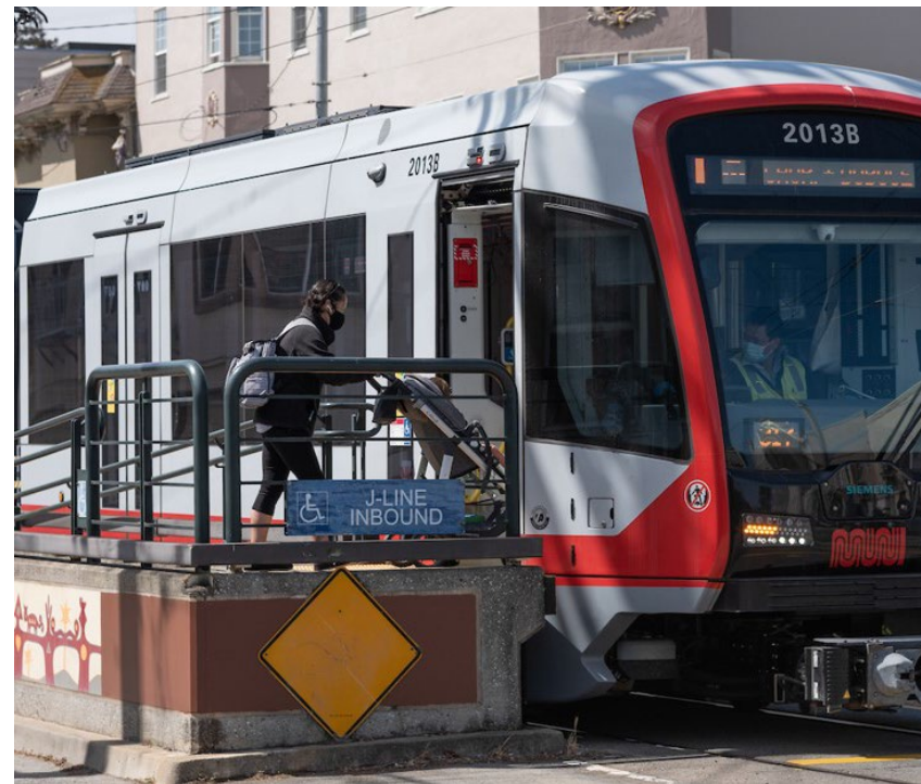
Existing mini-high ramp on the J Church
