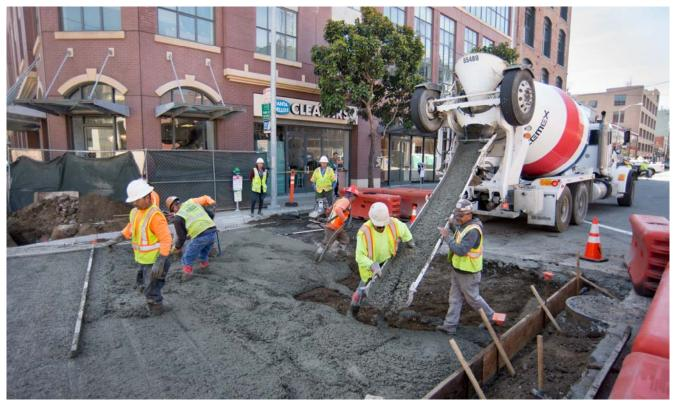
A new concrete road foundation slab is being poured at the southwest corner of 4th and Bluxome.
