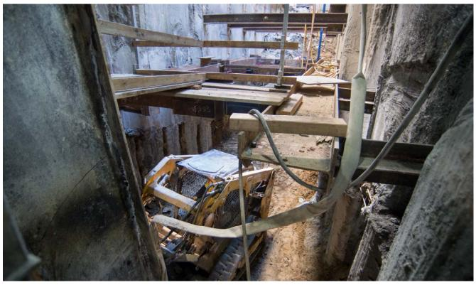
A bobcat fitted with a jackhammer is used to remove excess concrete from exterior tangent piles, comprising the station's outer walls. In this area on the east side of the station box at O'Farrell, workers are excavating a future emergency egress stairwell.
