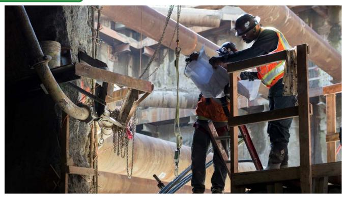
Two men review blueprints at the access portal between the station box and headhouse during invert rebar cage assembly.
