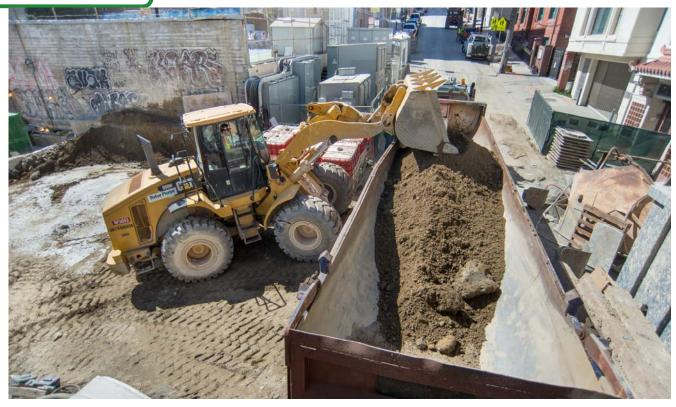
As material excavated below is brought to the surface of the headhouse, a loader collects it and distributes the load evenly in trucks for transport offsite.
