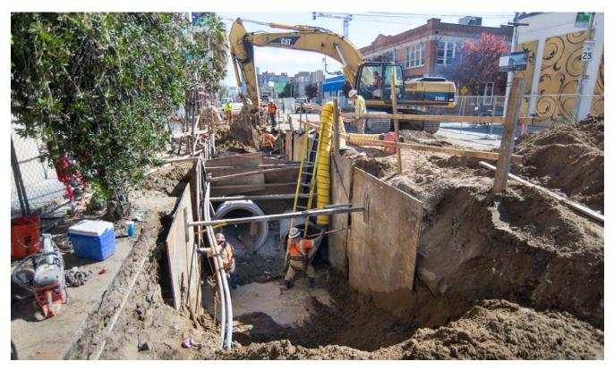
Two new sewer lines are visible on the east side of 4th south of Bryant, as workers continue to move up the street one section of pipe at a time.
