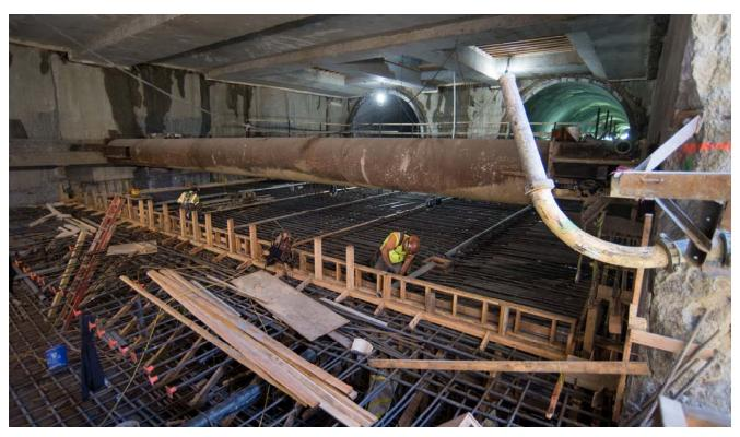
Workers install rebar at the south end of the station box's platform level, where it meets subway tunnels leading to and from the tunnel portal, only a block away.
