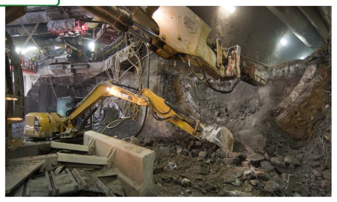
The faint outline of remaining tunnel segment pieces can be seen as it is removed during excavation of the left side drift for the north platform cavern.
