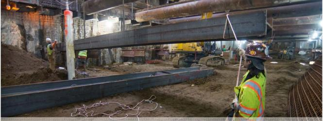
Workers wrangle and position a large steel I-beam just lowered into the station box from the surface.
