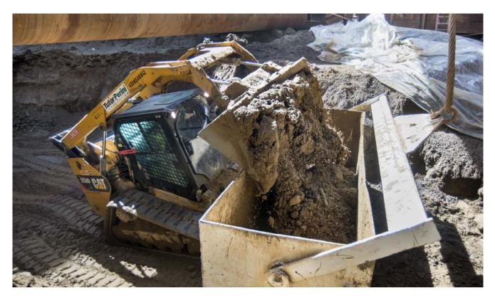
A bobcat dumps soil excavated from inside the station headhouse into a large steel bucket used to lift material to the surface for transport offsite.
