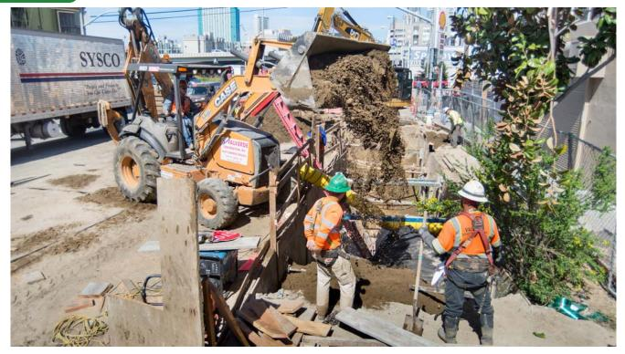
A backhoe brings a bucket of soil to bury newly-installed sewer pipes between Welsh and Bryant, on the east side of 4th.
