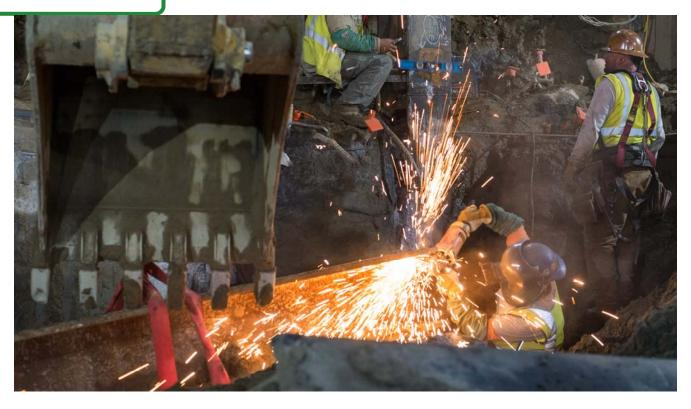
A metalworker cleans up the ends of a large steel I-beam for welding, which will be used as a bracket at the south headwall, near O'Farrell.
