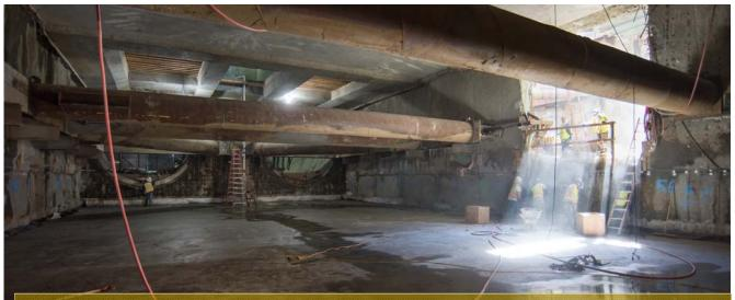
Light streams in the south end of the station box, where the initial "rat slab" for the remaining unconstructed portions of the platform level invert has been poured.
