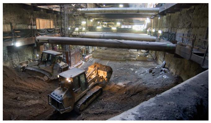
A bulldozer brings excavated material from inside the station cavern to a collection area at the south end of the headhouse. Here, the driver waits for the large steel bucket that brings material to the surface to be lowered.
