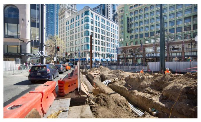
A bundle of utility conduits lay in a trench in a backfilled area on the south side of Ellis at Stockton and Market, where backfill and roadway restoration work are underway.
