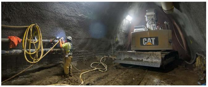
A worker checks the air pressure on a hose inside the left side drift of the north platform cavern, while a large excavator fitted with a grinding wheel works away nearby.
