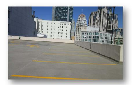
Improvements include a new waterproofing membrane with a 10-15 year life and comprehensive stall re-striping.
