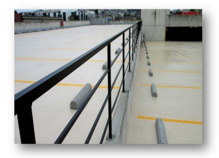
Improvements include a new waterproof membrane with a 10-15 year life as well as new stall striping, which included upgrade of the ADA-stall striping to meet current code.
