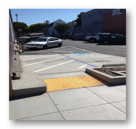
Improvements include upgrades to achieve ADA compliance to parking stalls and paths of travel, as well as complete repaving and upgrade of lighting fixtures.
