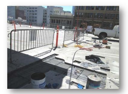
Improvements include targeted spalling repairs followed by installation of a new waterproofing membrane with a 10-15 year life.
