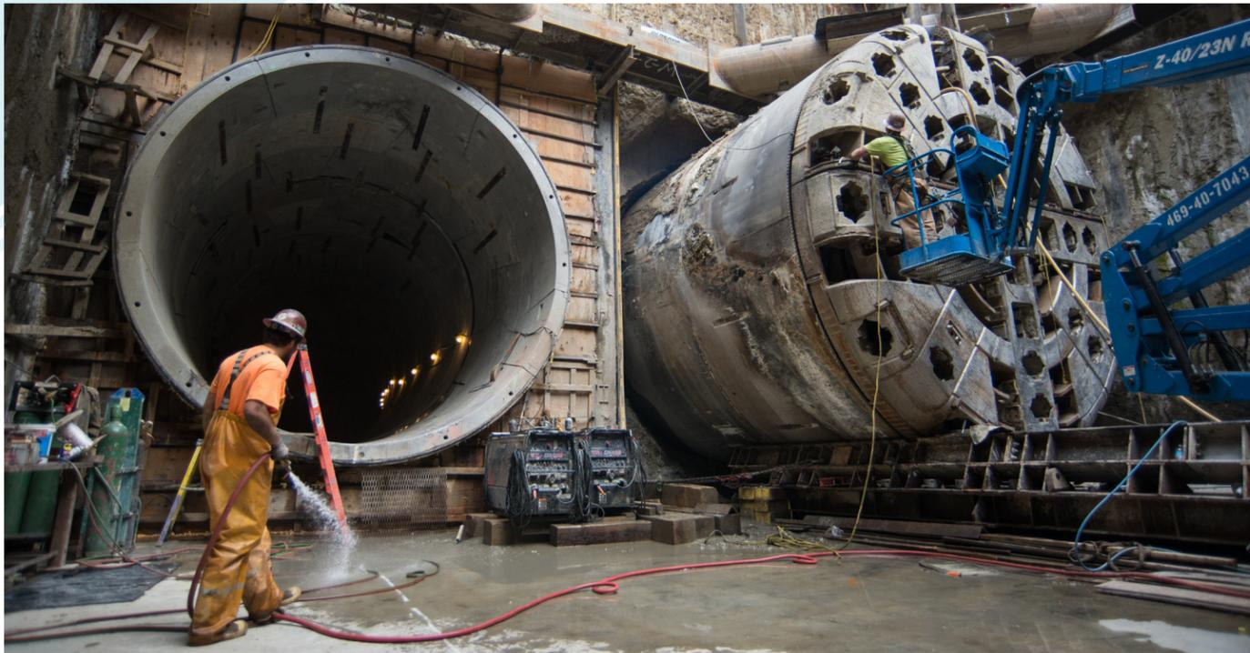
At the bottom of the former North Beach retrieval shaft, TBM Mom Chung can be seen being removed from the southbound tunnel while a worker keeps the site clean.
