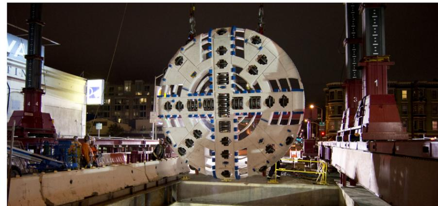
Lowering TBM Big Alma's cutterhead into the launch box
