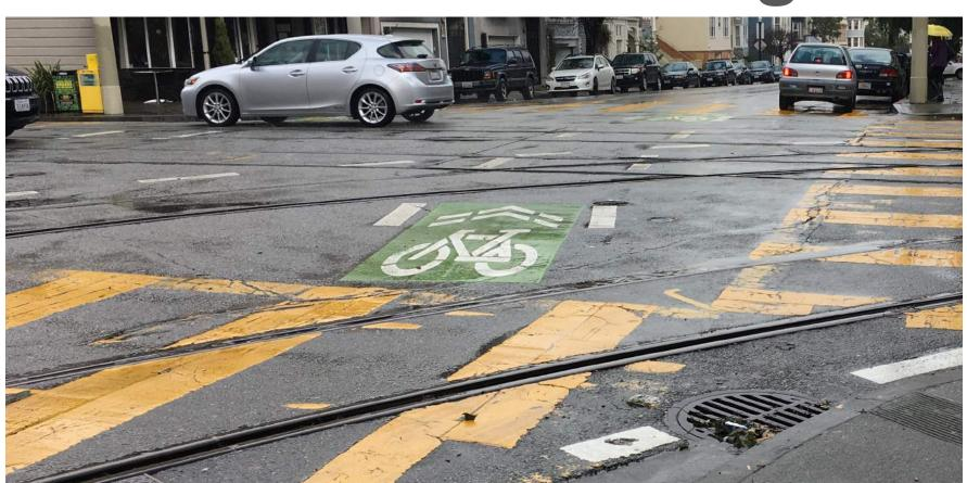
In 2012, SFMTA added markings on the pavement to guide cyclists on a recommended path of travel through the intersection. The markings are intended to encourage cyclists to cross the tracks at a better angle. These markings were upgraded in 2014.
