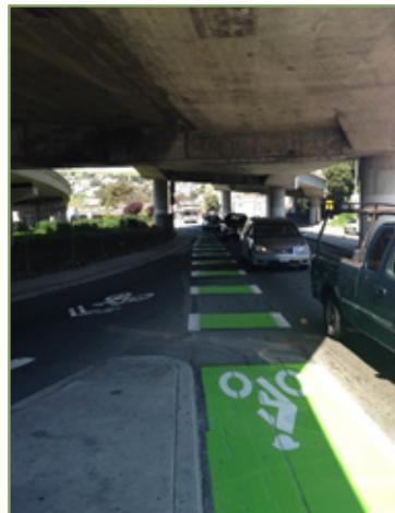
Additional bikeway striping at merging locations increases visibility of bicyclists, adds clarity to existing bicycle pavement markings, and clearly defines where vehicles should be expected to merge across the bike lane.
