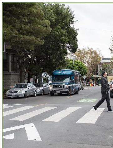
Similar to speed humps, but with a flat middle portion that can be used by pedestrians. Speed tables lower vehicle speeds to 15-20 mph, encouraging safer driver behavior on Neighborway streets with higher bicycle volumes.
