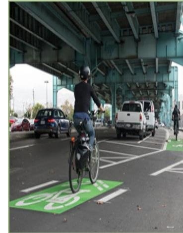
Pavement markings to guide bicyclists through an intersection and make the presence of bicyclists more visible to drivers. This treatment is especially helpful when a bikeway shifts laterally between one side of an intersection and the other.
