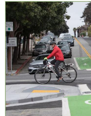
Diverters close off automobile access to a street while allowing space for people on bikes to pass through. Neighborways are most comfortable and safe when speeds and volumes are lower, and diverters are useful tool for lowering traffic volumes on local streets.
