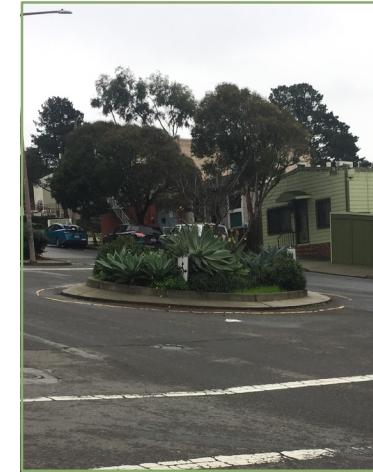
Traffic circles improve safety at intersections without adding a STOP sign, slowing vehicle speeds and reducing the number of conflicts at an intersection. Too many STOP signs can reduce compliance; traffic circles allow a better flow of traffic while keeping vehicle speeds low – perfect for a Neighborway.
