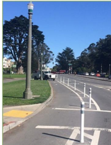
Vertical separation between the bikeway and the rest of the roadway, giving bicyclists greater comfort and safety. Vertical separation comes in a wide range of treatments.
