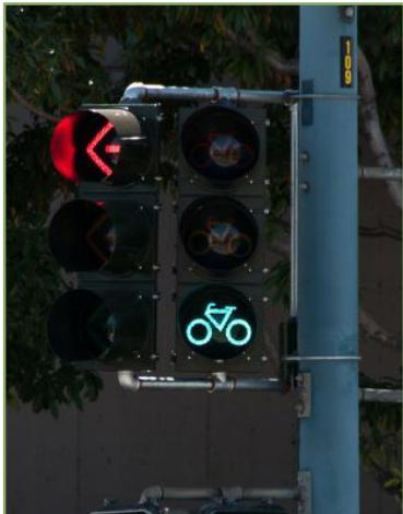
Bike traffic signals can be used in combination with protected intersections, when bike traffic flows need to be separated from turning movements, or to give bicyclists a leading interval when the lights change.
