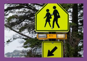
Rectangular Rapid Flashing Beacons are useractuated amber LEDs used at unsignalized intersections or mid-block crosswalks. In San Francisco, most RRFB's can be activated manually when pedestrians push a button. This evaluation collected data at two locations before and after the installation of RRFBs. We will be evaluating at least four other locations in 2019 to better understand the efficacy of this tool.
