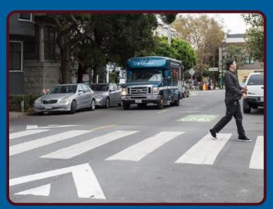
A Raised Crosswalks is a crosswalk that has been raised to the level of the sidewalk. This treatment prioritizes pedestrians and slows down vehicles when approaching the raised crosswalk.
