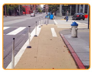
A Painted Safety Zone (PSZ) is an area around a pedestrian crossing where paint and plastic posts have been applied in the roadway. A PSZ helps to increase pedestrian visibility and reduces vehicle speeds while making turns at an intersection. In Bayview-Hunters Point, many intersection locations with perpendicular parking immediately adjacent to the crosswalk have been identified for a PSZ.
