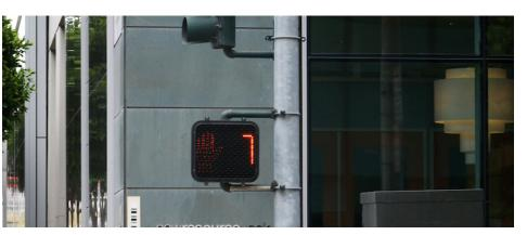
• Provides pedestrian the remaining time they have to cross the street before the traffic signal turns red.
