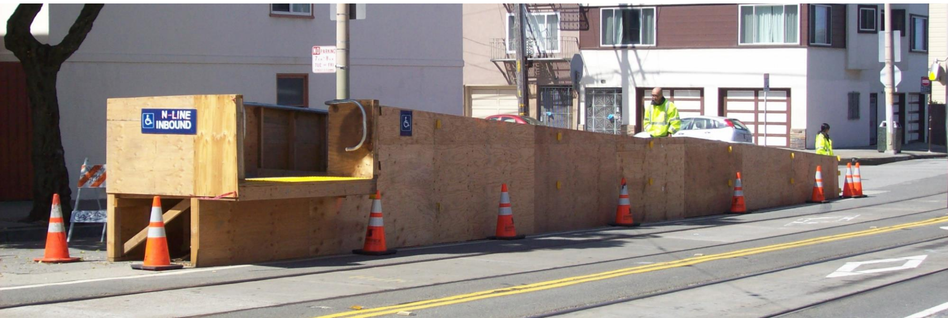
Example of a temporary accessible ramp
