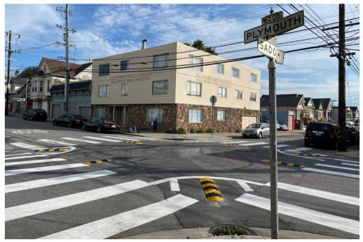
Figure 7: Example of exhibition driving deterrent treatments
