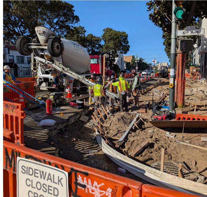
Bus bulb under construction at 6 th Ave outbound
