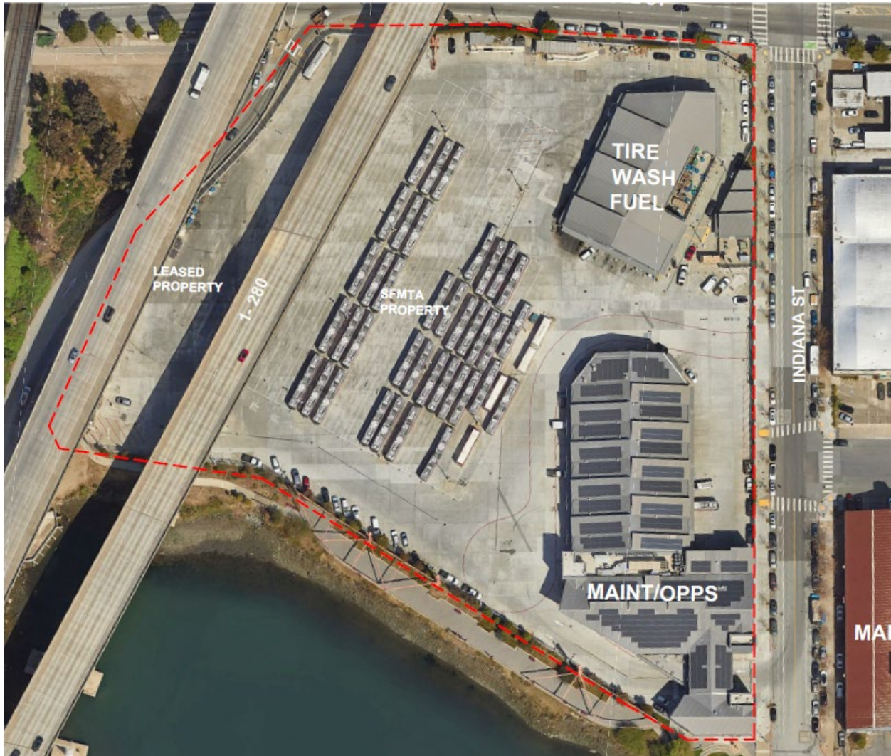
Figure 4-8. Islais Creek Yard - Existing Conditions (Aerial)
