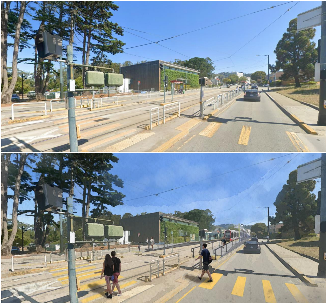
Figure 20: Photo illustration of possible upgrades to St. Francis Circle to provide level boarding
