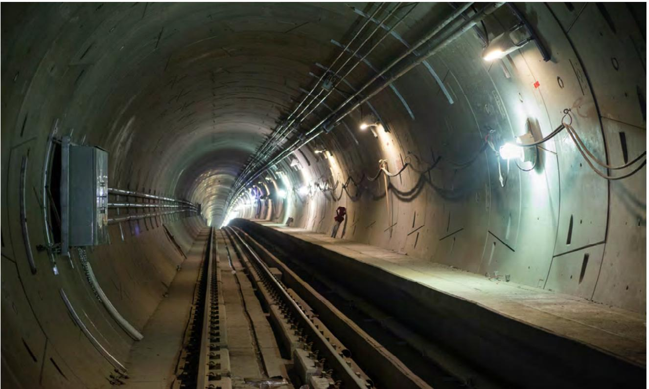
*New permanent LED lighting has been installed inside the northbound tunnel, as seen operating adjacent to temporary lighting, just south of the Chinatown track crossover cavern.*
