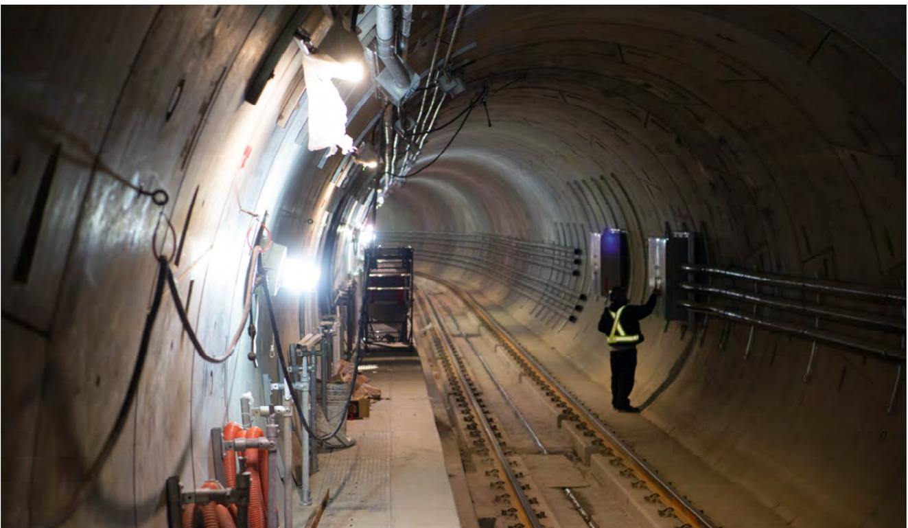
*Conduits for electrical, communications, and signaling systems, as well as initial walkway railing elements are being installed inside the northbound tunnel, seen here as it approaches the Market Street S-curve.*
