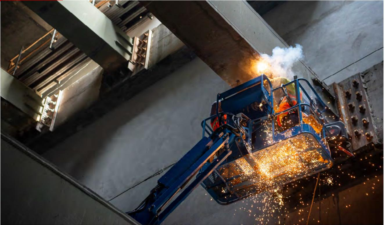
*Sparks fly as workers weld brackets to massive steel beams inside the Chinatown Rose-Pak Station entrance structure, where escalators and other interior elements are being installed.*
