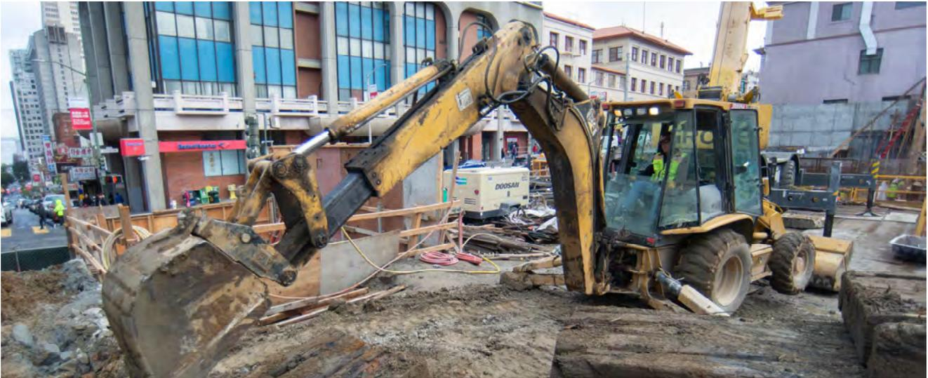
*A backhoe operator removes old cribbing used atop the north end of the Chinatown Station surface worksite.*
