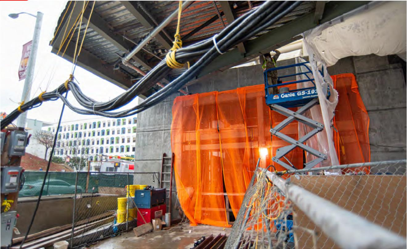
*Orange mesh covers future street level elevators down to the Yerba Buena/Moscone Station lobby, as a worker installs pipes for the fire suppression system above.*
