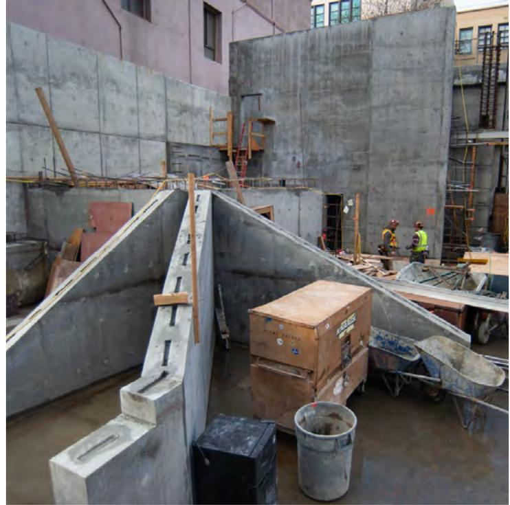
Reinforced concrete walls and foundation walls rise from the street-level surface slab at the future Chinatown Rose-Pak Station entrance.
