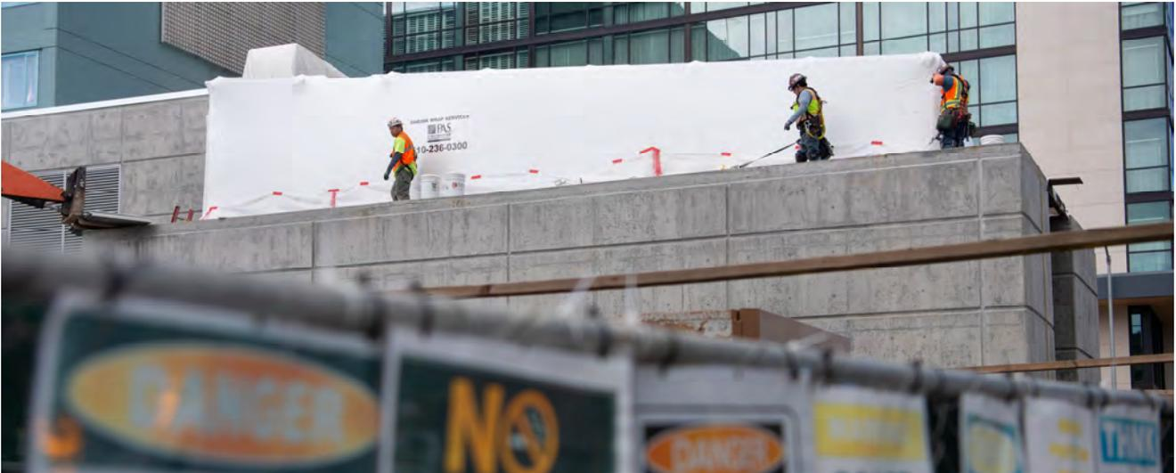
*Workers install plastic wrap and masking atop the Yerba Buena/Moscone Station headhouse entrance structure, currently under construction.*
