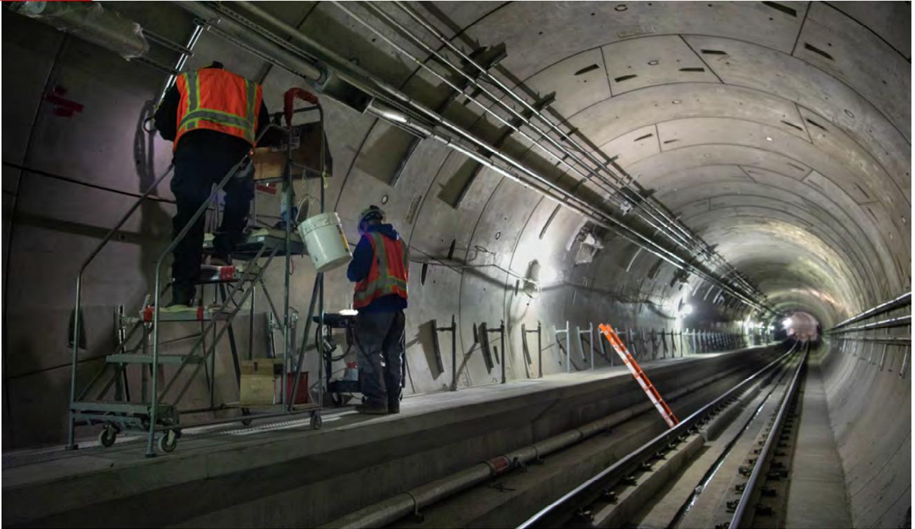
*Permanent lighting is being installed inside the northbound tunnel, just north of the Yerba Buena/Moscone Station platform.*
