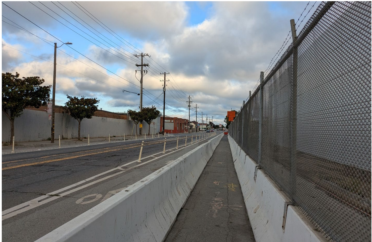
Evans Ave between Rankin Street & Quint Street, looking east:
