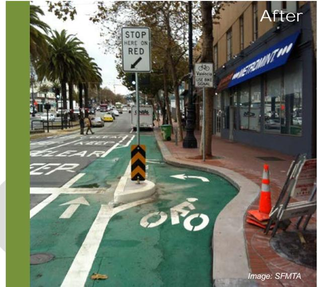
**After:** The SFMTA installed a bicycle signal and an innovative "bike bay" that allows people on bicycle to turn onto southbound Valencia Street via a protected crossing. This improvement closed a crucial gap in the bicycle network.
