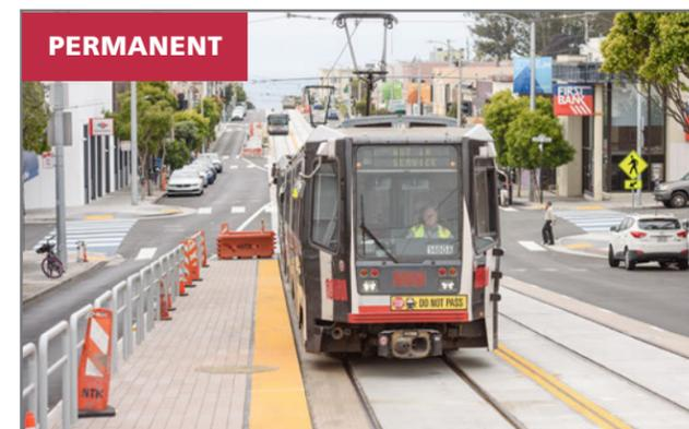
**Permanent transit boarding islands on Taraval:** Quick-build safety zones have been replaced with new permanent boarding islands made of concrete at all stops on Taraval Street.
